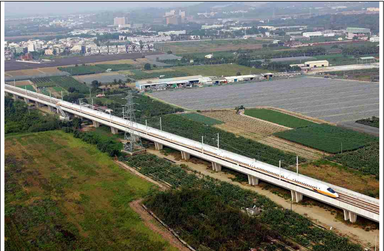
Fig. 1 Simply supported spans of 25 to 35 meter represent the most frequent structural scheme for most of the High Speed Rail bridges like Taiwan as shown in the picture
