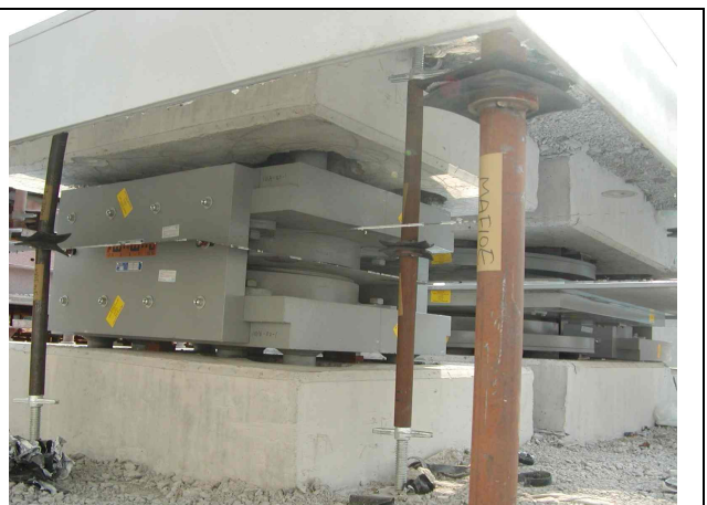
Fig. 11 Detail of the antilifting clamps utilized for the Taiwan High Speed Rail
