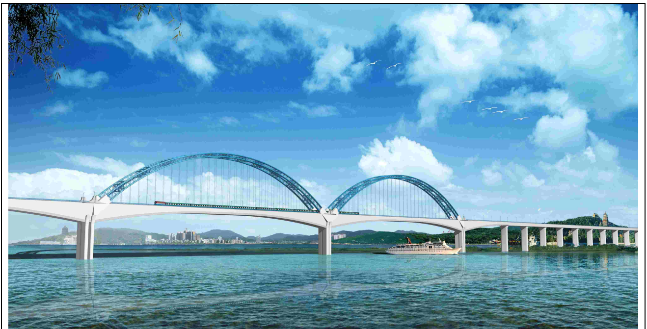
Fig. 4 An outstanding example of bow-string structure: the Yi-Chang bridge for the Chinese Rail System
