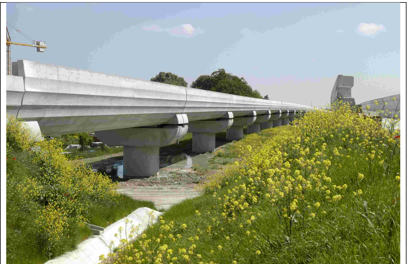
Fig. 2 The Modena viaduct of the Italian High Speed Rail. Simply supported spans of 35 meter for a total length of 18 km
