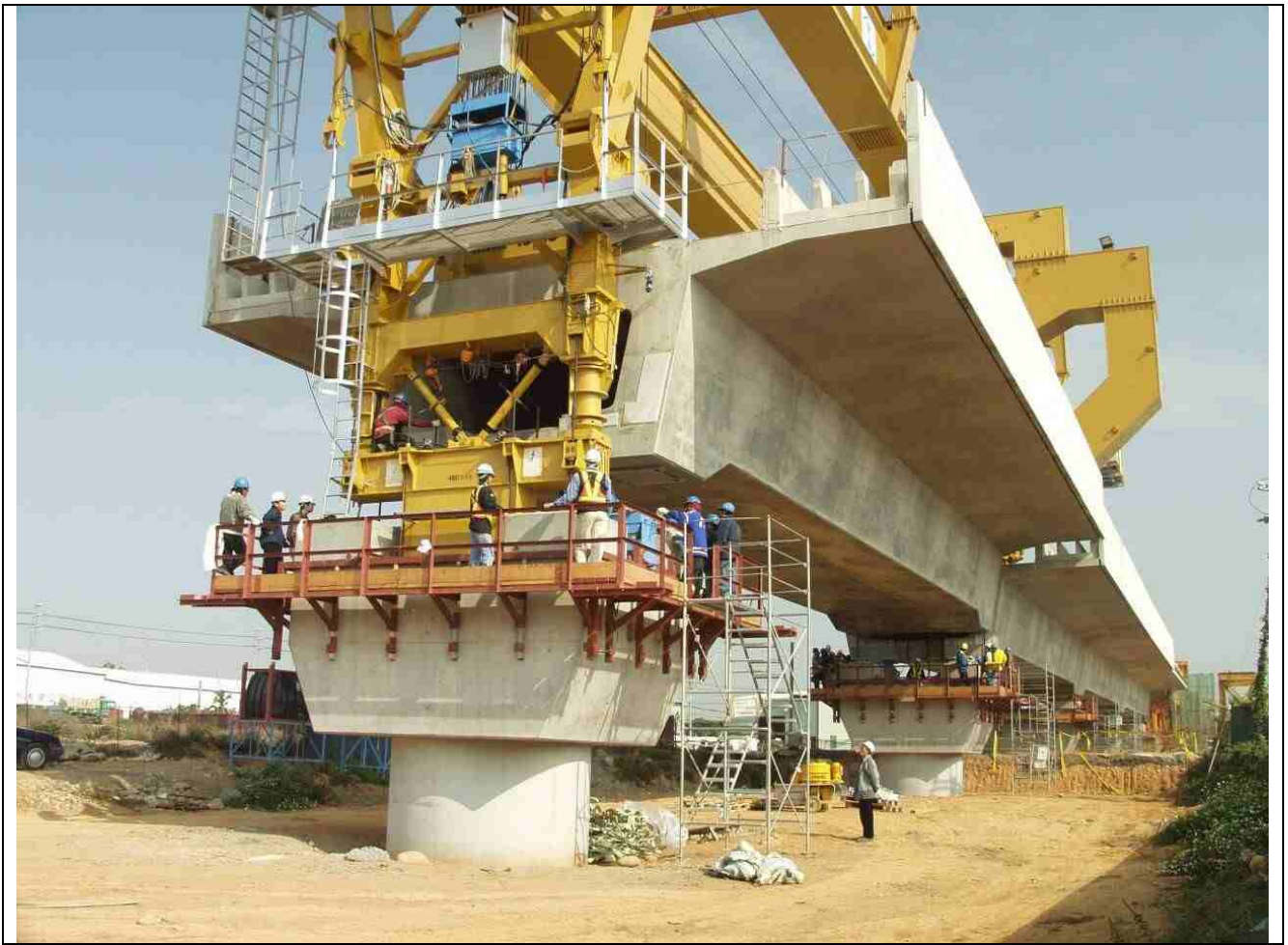
Fig. 18 The Taiwan High Speed Railway under construction
