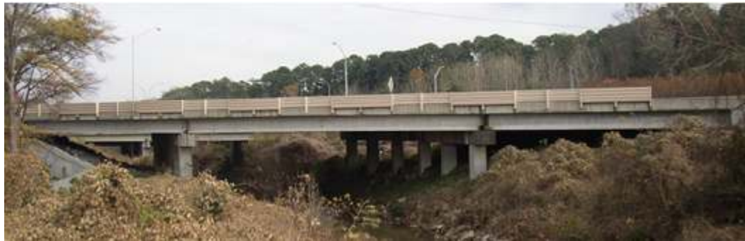
Figure 5.1 Picture of example MSC Steel Girder Highway Bridge (Nielson 2005).
