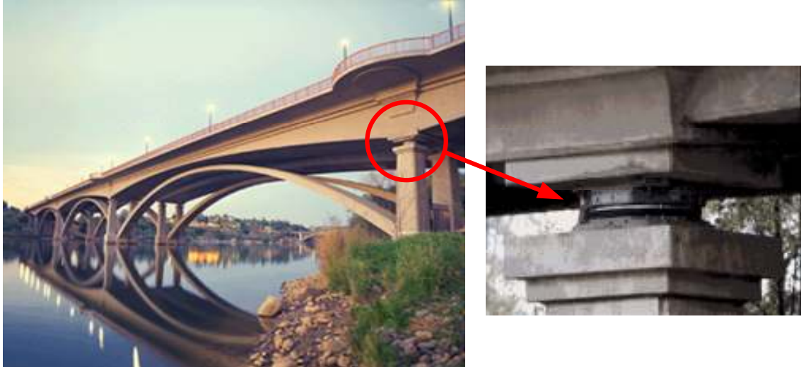
Figure 1.1 Typical seismic isolation example in the American River Bridge at Lake Natoma in Folsom, California (courtesy of Earthquake Protection Systems, Inc.).
