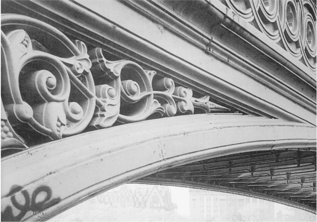
FIGURE 67.7 Bow Bridge in Central Park, New York, is the oldest surviving wrought-iron bridge in the United States, built in 1862. It has the longest span, 26.5 m, of five ornately decorated bridges in the park, all designed by Calvert Vaux and Jacob Wrey Mould. (Courtesy of American Society of Civil Engineers.)
