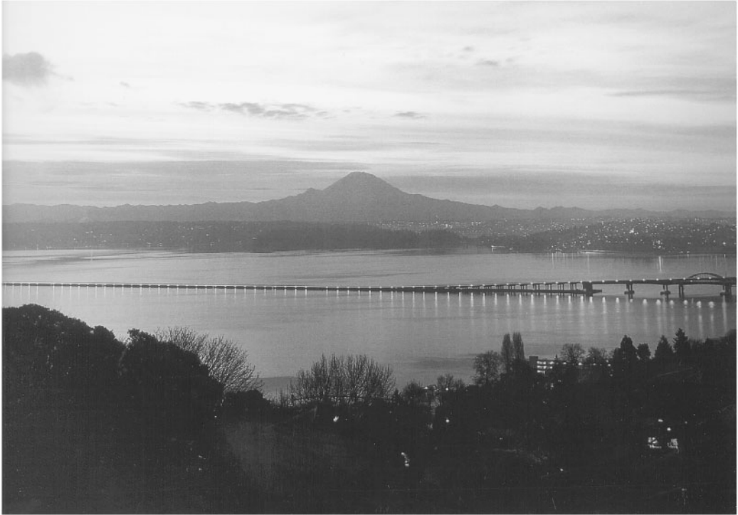
FIGURE 67.38 The 2377-m-long Lacey V. Murrow Floating Bridge across Lake Washington near Seattle is composed of hollow concrete pontoons. The depth of water, 45.7 m, precludes piers, but there are some bridge spans over shallow water near the shore that can pass small vessels. It was designed by Charles Andrew and Clark Elkrige in 1940. The bridge is listed on the National Register of Historic places. (Courtesy of American Society of Civil Engineers.)
