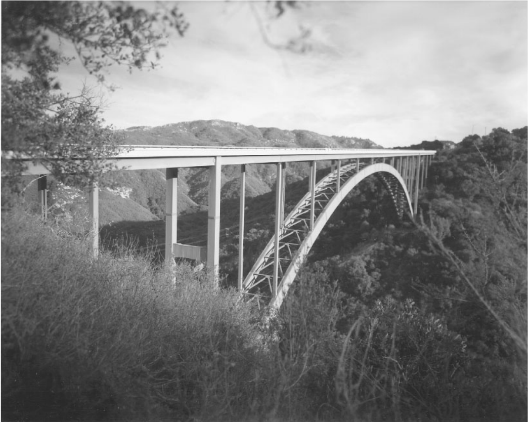
FIGURE 67.14 The Cold Springs Canyon steel plate girder arch, in Santa Barbara County, California, is the longest arch span at 213.4 m, and a rise of 121.9 m. The bridge has won a Lincoln Foundation welding award, American Institute of Steel Construction beauty award, and the Governor's Design Award. Built in 1963, it was designed by the California Division of Highways, Marv Shulman, design engineer. (Courtesy of California Department of Transportation.)
