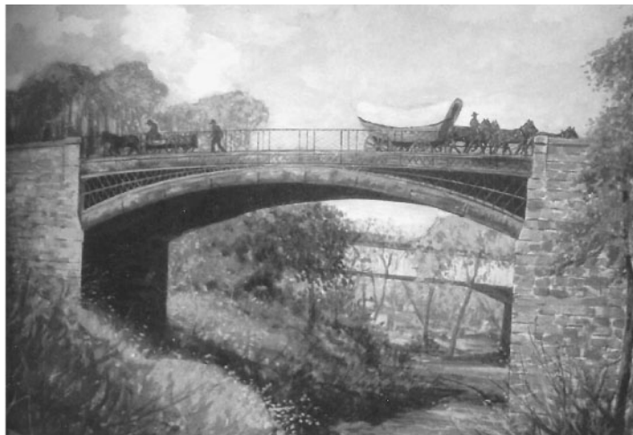
FIGURE 67.6 Dunlap's Creek Bridge, built in 1839, is the first iron bridge in the United States. It was built for the National Cumberland Road, at Brownsville, Pennsylvania, by Captain Richard Delafield of the Army Corps of Engineers. The bridge is still in service today. (Courtesy of Federal Highway Administration.)
