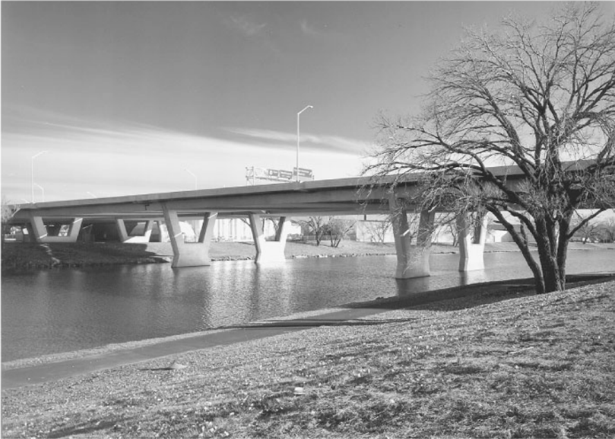
FIGURE 67.42 Kellogg Central Business District Viaduct in Wichita, Kansas, designed by Howard Needles Tamman Bergendoff, won a Portland Cement Association award in 1996. (Courtesy of Howard Needles Tamman Bergendoff.)
