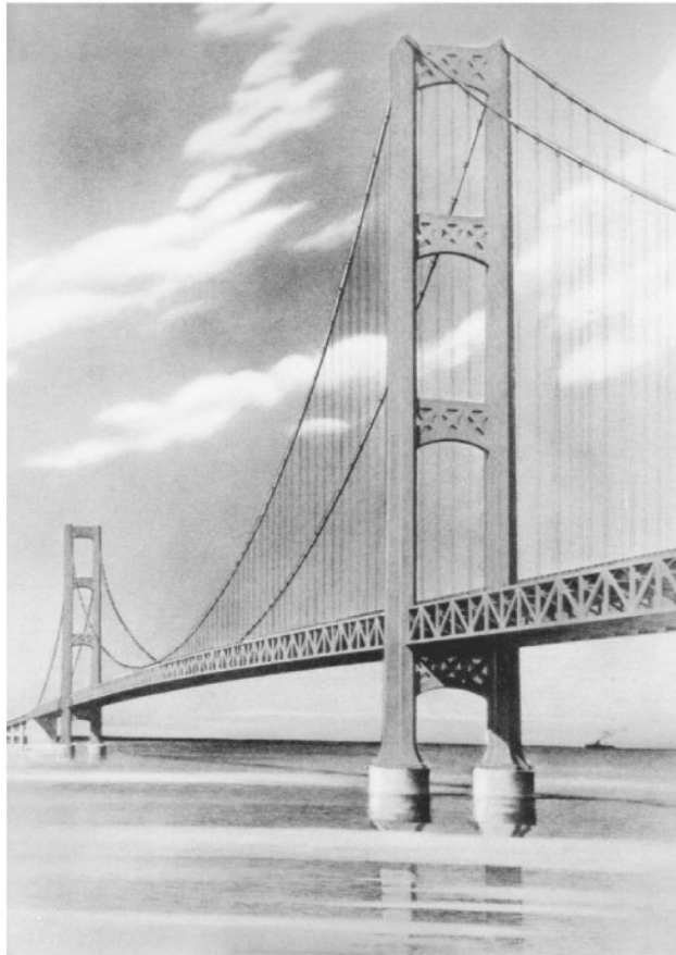
FIGURE 67.34 The Mackinac Straits Bridge was the winner of the 1958 American Institute of Steel Construction's Artistic Bridge Award and several gold medals. Its design provided a level of aerodynamic stability never before attained in a suspension bridge. It has a main span of 1158 m. It was designed by David Steinman and is owned by the Mackinac Bridge Authority in northern Michigan. (Courtesy of David Steinman.)
