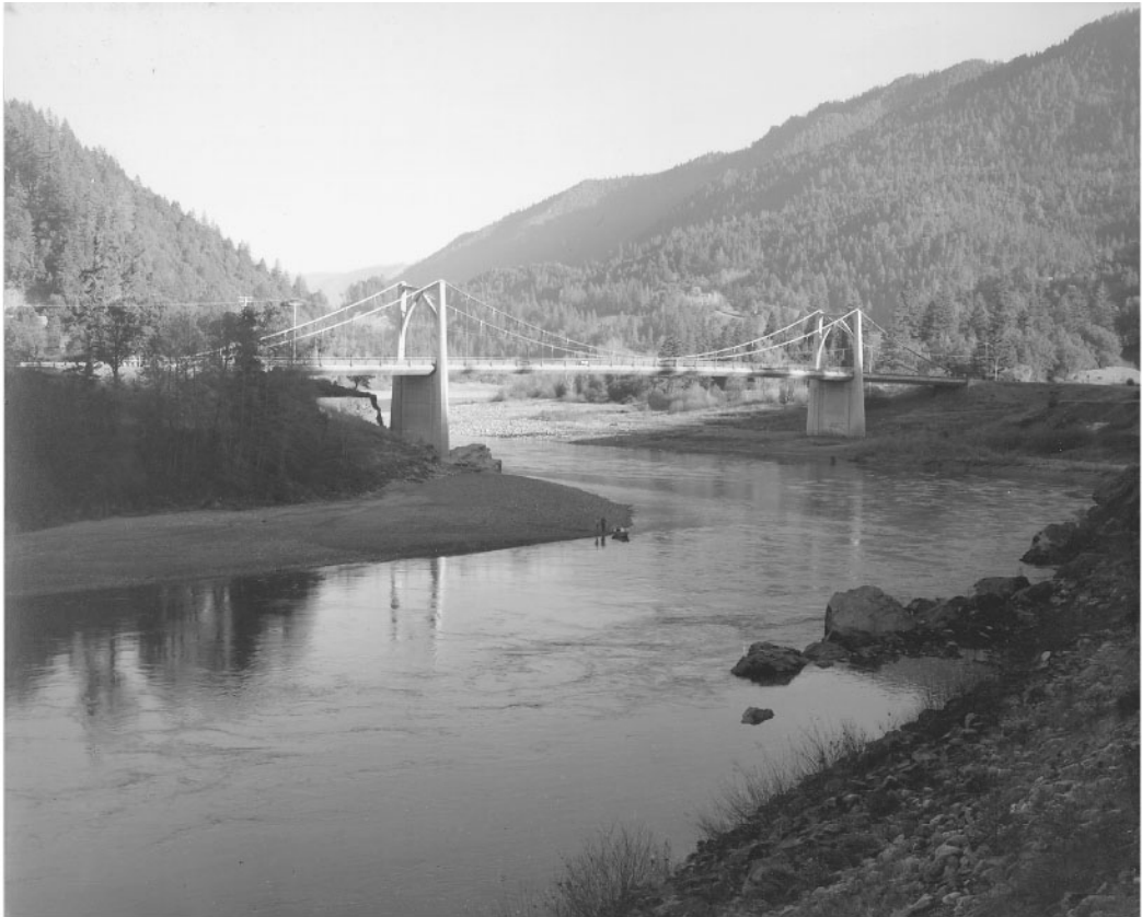
FIGURE 67.47 The Klamath River crossing at Orleans in Northern California is a picturesque setting on a back road. There have been seven structures at this site, one burned and five have been washed away during major floods. The current steel box girder suspension span has lasted longer than any of its predecessors. Built in 1967, it was designed by Bert Bezzone of the California Division of Highways. (Courtesy of California Department of Transportation.)
