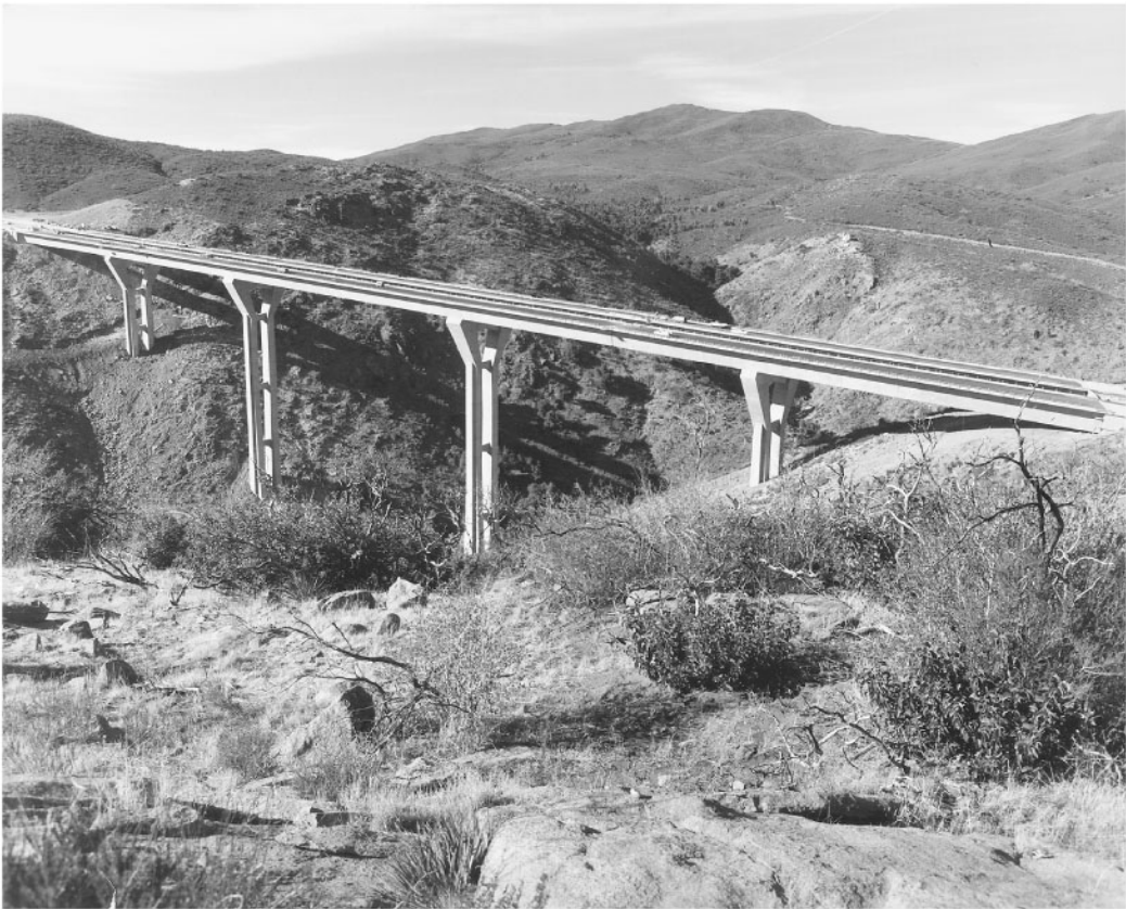
FIGURE 67.50 The California Department of Transportation experimented with and built its only segmental bridge, on Interstate Route 8 over Pine Valley in San Diego County in 1974. Bert Bezzone was the design engineer. The bridge received an American Society of Civil Engineers award in 1974. (Courtesy of California Department of Transportation.)
