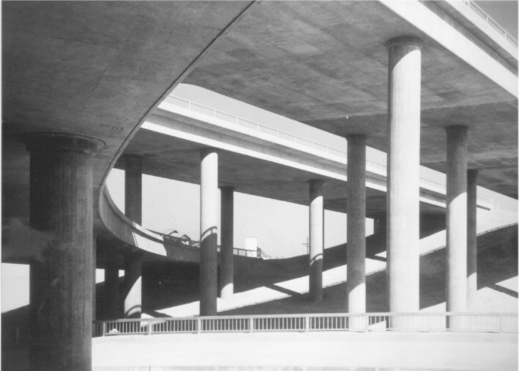
FIGURE 67.39 The Four Level Interchange in downtown Los Angeles, built in 1950, is the first multilevel interchange of two freeways. It is a reinforced concrete box girder, a type developed by, and to become the hallmark of, the California Division of Highways. (Courtesy of California Department of Transportation.)
