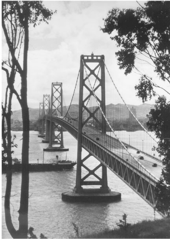
FIGURE 67.32 The west span of the San Francisco–Oakland Bay Bridge is really two suspension bridges end to end with a central anchorage between the two. It is the only double-suspension bridge in the world. Opened in 1936, it is owned by the California Department of Transportation and designed by its predecessor, the California Division of Highways, Charles Andrew, Chief Bridge Engineer. (Courtesy of California Department of Transportation.)
