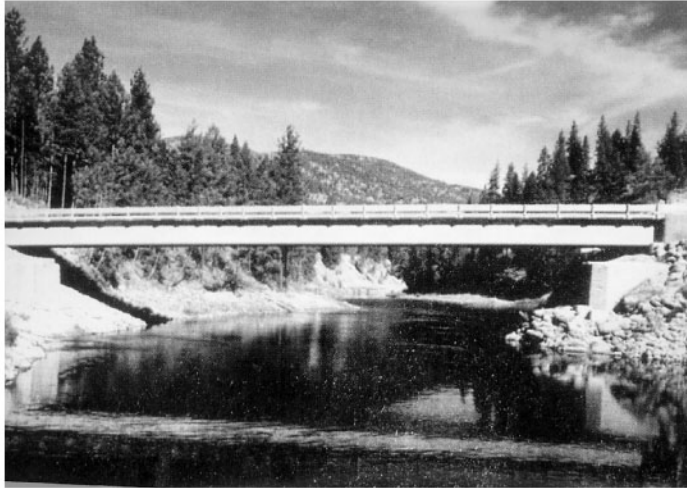
FIGURE 67.28 Rockcut Bridge, owned by Stevens and Ferry Counties, earned a Portland Cement Association design award in 1997. The designer was Nicholls Engineering. (Courtesy of Portland Cement Association.)
