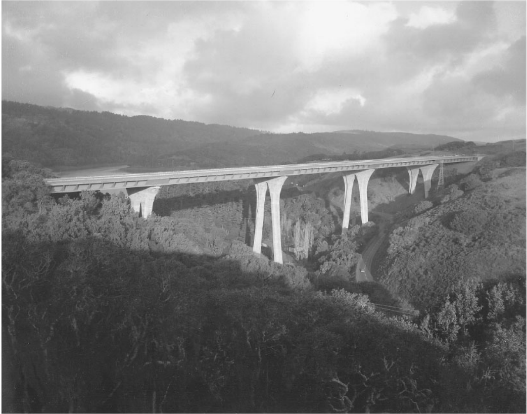
FIGURE 67.45 The Eugene A. Doran Memorial (San Mateo Creek–Crystal Springs Reservoir) Bridge is a prize-winning bridge in a park setting. Sloping exterior fascia plates provide web stiffening and aesthetic treatment. This welded plate steel girder bridge, built in 1970, was designed by Bob Cassano of the California Division of Highways. (Courtesy of California Department of Transportation.)
