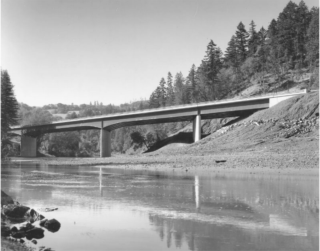
FIGURE 67.43 The South Fork of the Eel River Bridge in Northern California exemplifies the virtues of composite steel structures. This 1958 bridge won an AISC award that year. (Courtesy of California Department of Transportation.)
