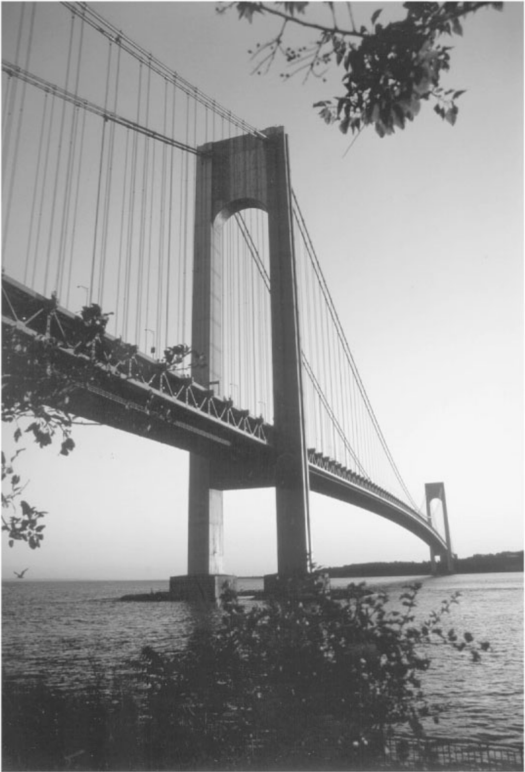
FIGURE 67.35 The Verrazano Narrows Bridge, in New York City, has the longest span, 1298 m, of any bridge in America. Designed by Amman and Whitney, it was opened in 1964. (Courtesy of Metropolitan Transportation Authority, New York.)
