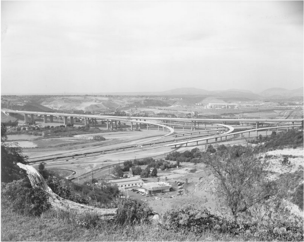
FIGURE 67.40 Mission Valley Viaduct sweeps Interstate Route 805 over the San Diego River floodplain in southern California. (Courtesy of California Department of Transportation.)
