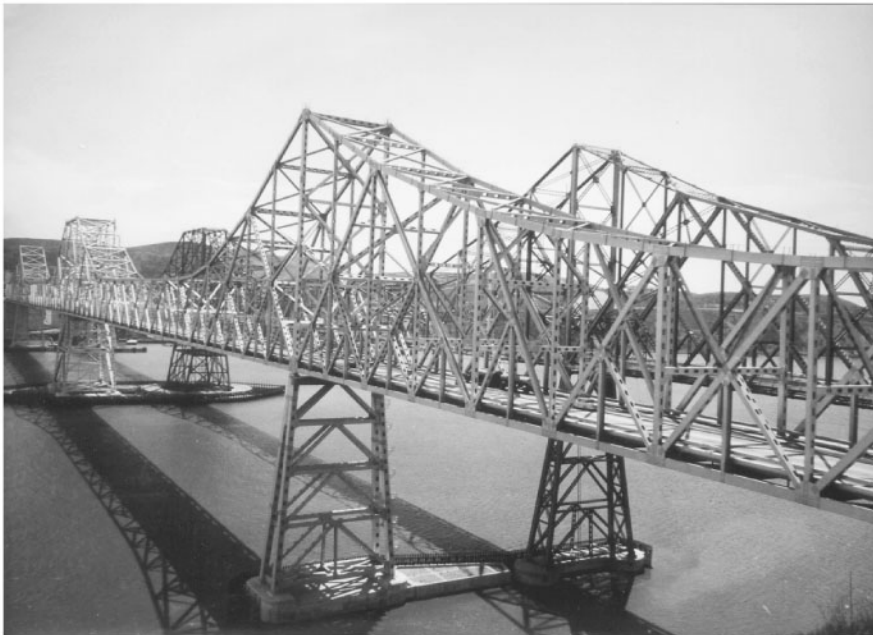
FIGURE 67.17 The Carquinez Straits Bridge in California, built by the American Toll Bridge Company as a private toll bridge in 1927, is an example of a cantilevered truss with eye bar tension members. A parallel twin using welded hybrid high-strength steels was designed and built in 1954 by the California Division of Highways, Roger Sunbury, engineer. Steel truss bridges are considered by many to be ugly. Carquinez is not one of the worst examples, but when a candidate bridge architect interviewing for the California Department was shown a picture of the twin spans and asked for comments, he answered, “Why make the same mistake twice?” He got the job as Chief Bridge Architect. (Courtesy of California Department of Transportation.)
