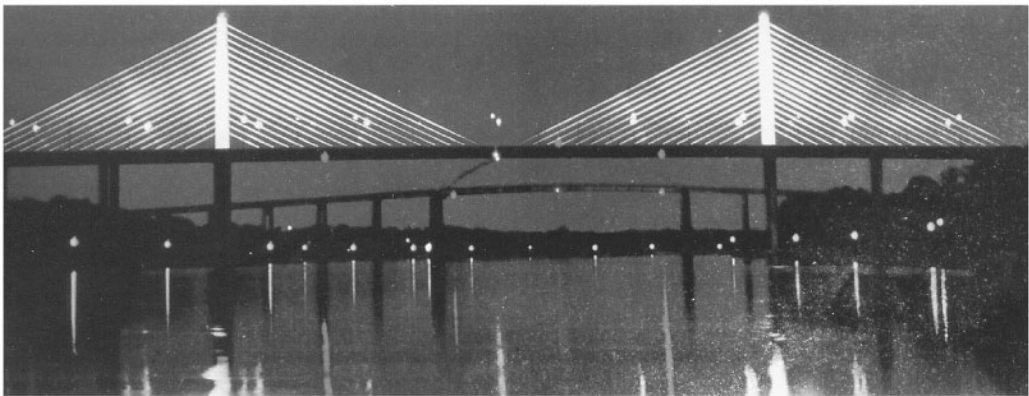
FIGURE 67.53 The Chesapeake and Delaware Canal Bridge owned by Delaware Department of Transportation was designed by Figg Engineering. It received an Excellence in Design Award in 1996. (Courtesy of Figg Engineering.)
