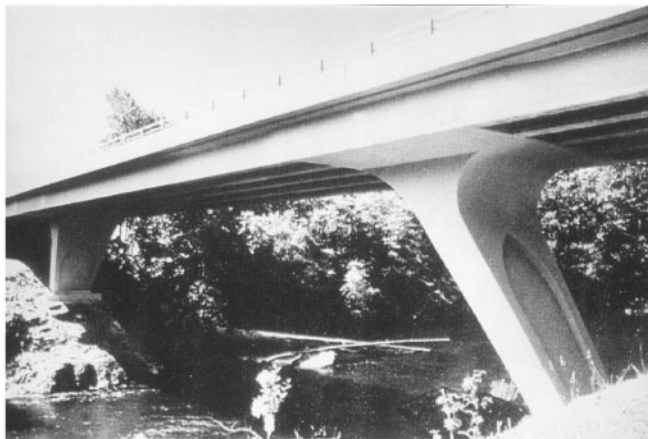
FIGURE 67.29 The North Santiam (Gates) Bridge, in Marion County, Oregon, earned a Portland Cement Association design award in 1997. It was designed by the Oregon Department of Transportation. (Courtesy of Portland Cement Association.)
