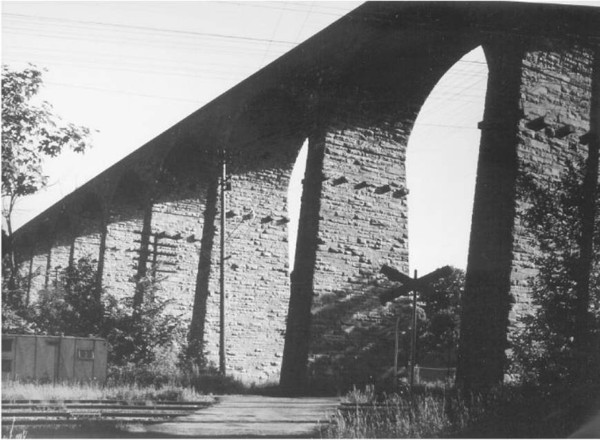
FIGURE 67.8 Starrucca Viaduct, built in the form of the ancient Roman aqueducts, was designed by James Kirkwood for the New York and Erie Rail Road in 1848. It is located over the Starrucca Creek plain at Lanesboro, Pennsylvania. This was the first bridge to use a concrete foundation. This bridge is still in service. (Courtesy of American Society of Civil Engineers.)
