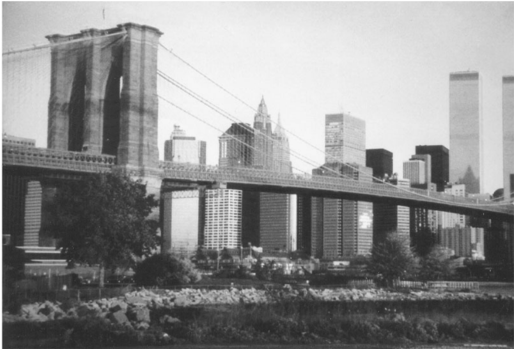
FIGURE 67.31 The Brooklyn Bridge is probably the best known of the classic U.S. bridges. It is one of the early uses of wire rope, being a combination suspension and cable-stayed span. Designed and built in 1883 by John and Washington Roebling for the City of New York. (Courtesy of American Society of Civil Engineers.)
