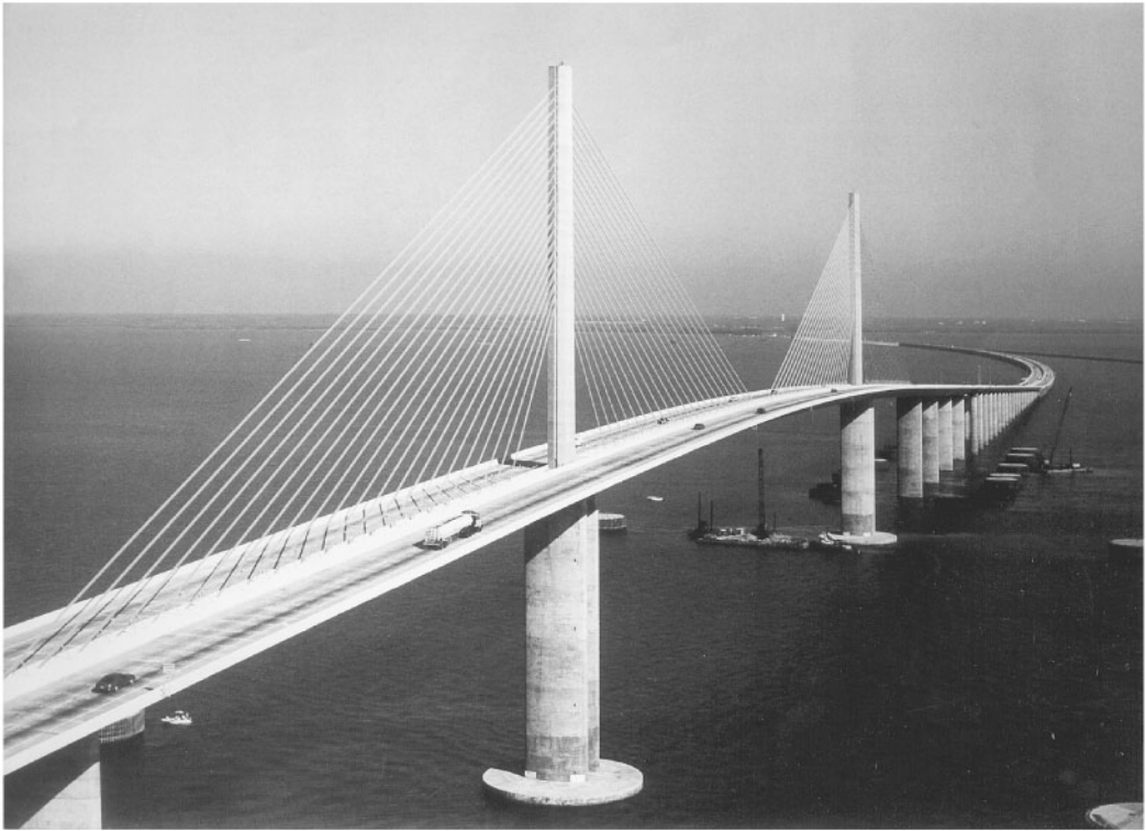
FIGURE 67.52 The new cable-stayed Sunshine Skyway, built in 1987, clearly a signature bridge, makes a bright statement over the entrance to Tampa Bay, Florida. This structure by Figg Engineering replaced the former Sunshine Skyway truss brought down by an errant barge that weighed more than that bridge. The new piers are protected by caissons as big and heavy as that barge. (Courtesy of Figg Engineering.)
