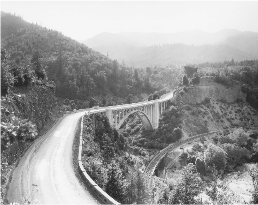
FIGURE 67.23 Harlan D. Miller (Dog Creek) Bridge is an example of state-of-the-art bridge development by the State of California under Bridge Engineer Harlan D. Miller in 1926. The State Legislature named the bridge in his honor for the great strides he accomplished with state bridges. Miller died only a week after receiving the honor, so the bridge became the Harlan D. Miller Memorial Bridge. (Courtesy of California Department of Transportation.)
