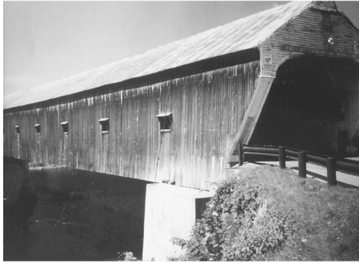
FIGURE 67.5 The Cornish–Windsor Covered Bridge is a two-span town-lattice truss crossing the Connecticut River between Cornish, New Hampshire and Windsor, Vermont. Built in 1866 it is the longest covered bridge, 140.2 m, in the United States. It has been designated a National Civil Engineering Landmark by the American Society of Civil Engineers. (Courtesy of American Society of Civil Engineers.)
