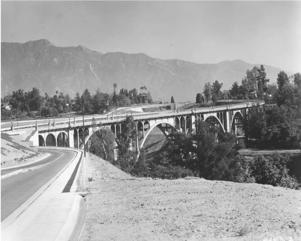
FIGURE 67.21 The Colorado Street Bridge over the Arroyo Seco in Pasadena, California, is the highest scoring bridge for historical significance in the state. The main span is 46.6 m with a height of 45.7 m. The structure is highly adorned with Beaux Art ornamentation. It was designed in 1912 by John Waddell, the “Dean” of American bridge engineering. The bridge served the famed Route 66 for many years. Seismic retrofitting was a challenge in trying to maintain the bridge’s historic aesthetic features. (Courtesy of California Department of Transportation.)
