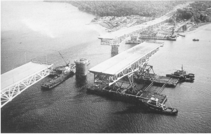
FIGURE 67.37 The double-swing span George P. Coleman Bridge over the York River in Yorktown, Virginia, was recently widened. To minimize impacts on heavy traffic flows, new truss sections were built in dry dock and floated into place as the old were floated out. The replacement designed by Parsons, Brinckerhoff, Quade and Douglas won the 1997 George P. Richardson Medal for outstanding achievement. (Courtesy of Parsons Brinckerhoff.)
