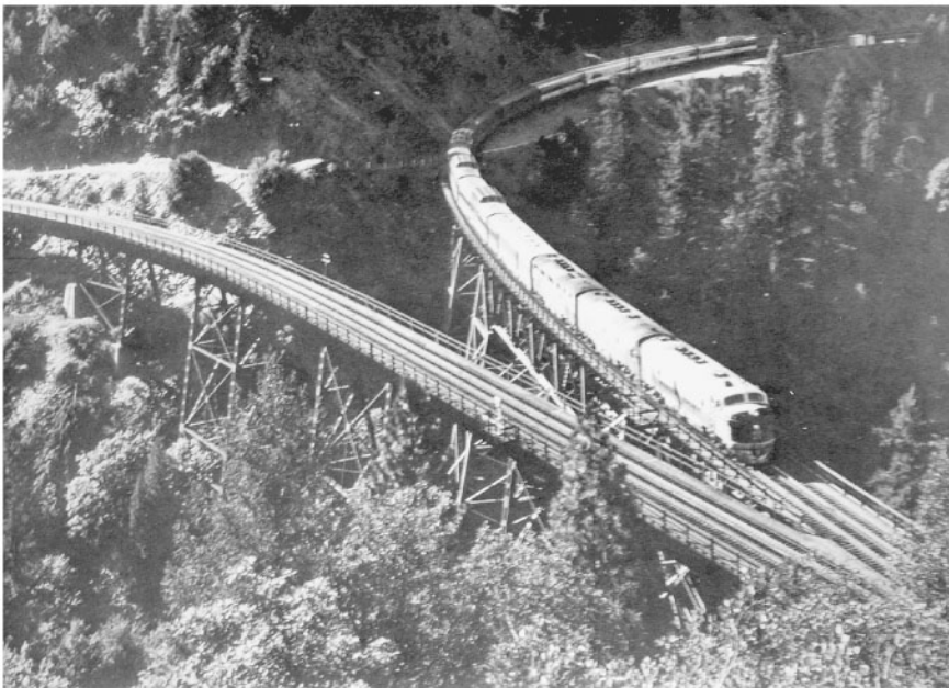
FIGURE 67.11 Keddie Wye is a unique steel tower trestle built by the Union Pacific Railroad in California's rugged Feather River Canyon in 1912. The wye trestle emerges from a tunnel in the south wall of the canyon splitting rail traffic over the river; one leg heads north to meet with the Burlington Northern Railroad and the other is the main line heading east toward Chicago. (Courtesy of the Feather River Rail Society.)
