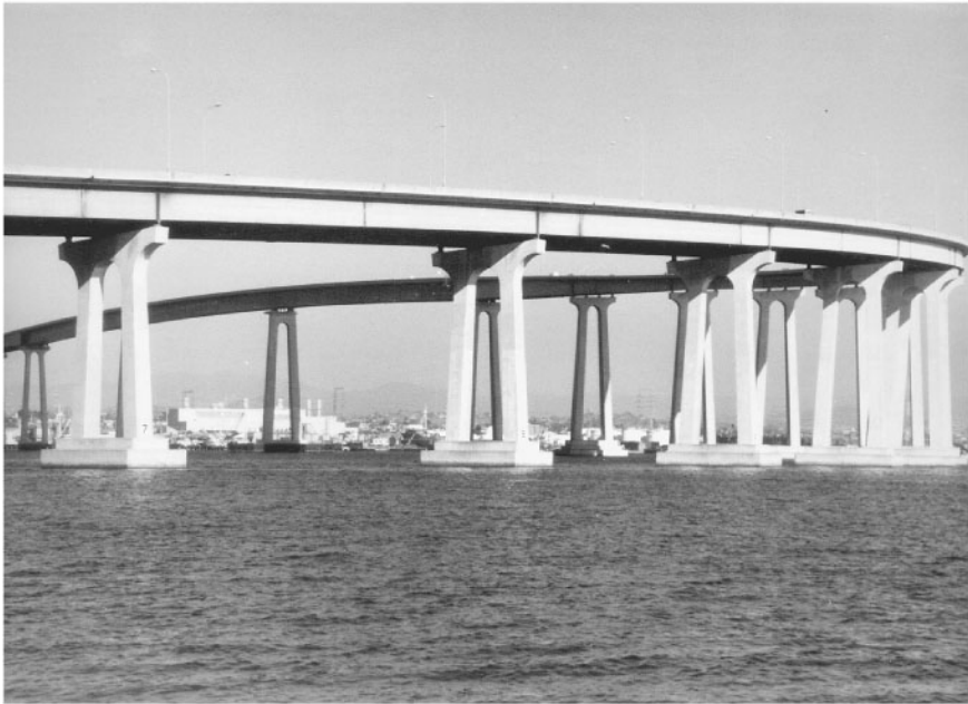
FIGURE 67.49 The Coronado Island Bridge over San Diego Bay in Southern California is a steel box girder. It earned an AISC award in 1970. It was designed by the California Division of Bay Toll Crossings. (Courtesy of California Department of Transportation.)
