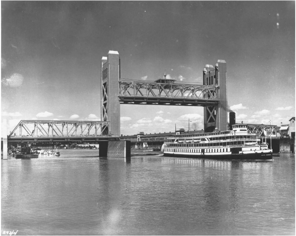
FIGURE 67.36 The Tower Bridge in Sacramento earned an AISC design award in 1936, the year in which it was built. This unique lift span is clad in steel plate to cover the moving parts. It was designed by Leonard Hollister of the California Division of Highways. (Courtesy of California Department of Transportation.)
