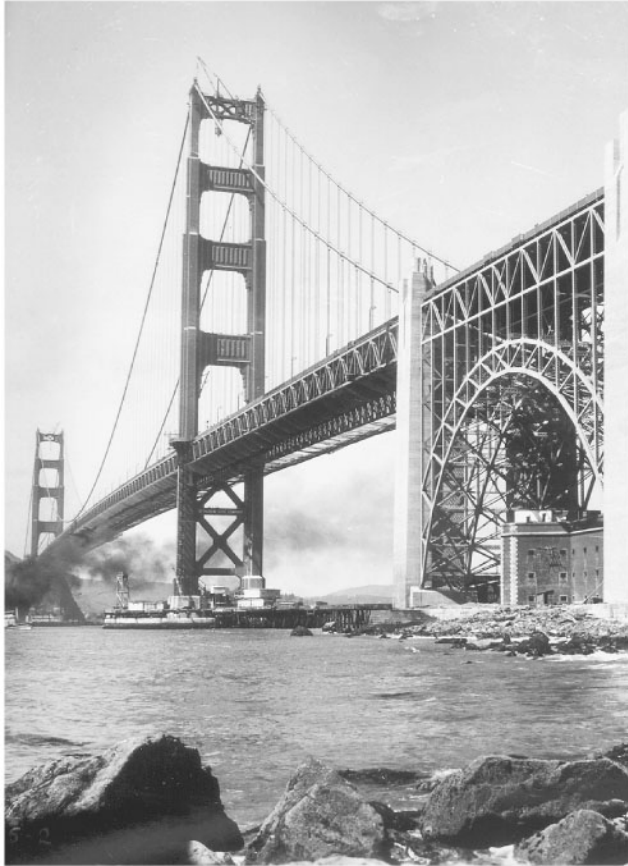
FIGURE 67.33 The Golden Gate Bridge is one of the best-known landmarks in the United States. It spans the entrance to San Francisco Bay. It held the longest span, 1280 m, record for 27 years. Designed and built in 1937 by Charles B. Strauss. It is owned by the Golden Gate Bridge, Highway and Transportation District. (Courtesy of California Department of Transportation.)
