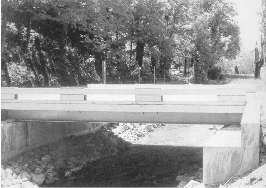
FIGURE 67.54 Laurel Lick Bridge is the second all-composite bridge to be completed. It is owned by the West Virginia Department of Highways and was built experimentally in conjunction with West Virginia University, in 1997. (Courtesy of West Virginia Department of Highways.)
