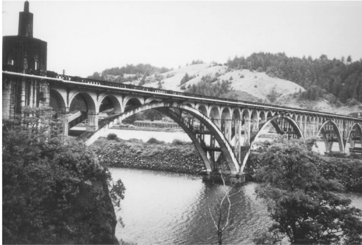
FIGURE 67.25 Conde McCullough, of the Oregon State Highway Department, designer of the two bridges shown in Figures 67.25 and 67.26 , gained fame as the designer of several landmark bridges on the Oregon Coast Highway. The Rogue River Bridge at Gold Beach, Oregon, is a typical open spandrel concrete arch. The monumental spires at the abutment piers are a McCullough trademark. Both of these bridges were built in 1932. (Courtesy of Oregon Department of Transportation.)
