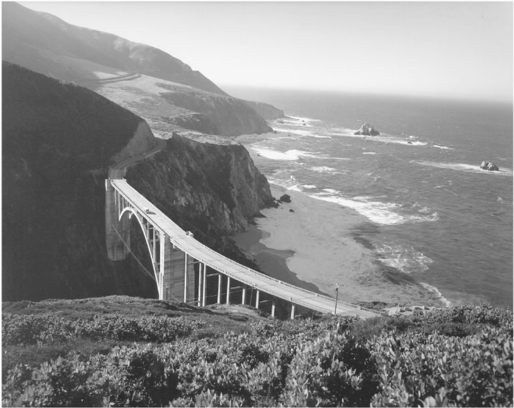
FIGURE 67.24 Bixby Creek Bridge on the Monterey Coast in California is one of the most picturesque and photographed bridges in California. This Monterey Coast Highway was the first designated Scenic Highway in California, in 1961. The route is also the first to be designated an All American Road. Built in 1932, it has a main span of 109.7 m and is 79.2 m above the streambed. Construction required 26 stories of falsework. It was designed by Harvey Stover of the California Division of Highways. Seismic retrofitting is complicated due to aesthetic restrictions established by historical preservation codes. (Courtesy of California Department of Transportation.)
