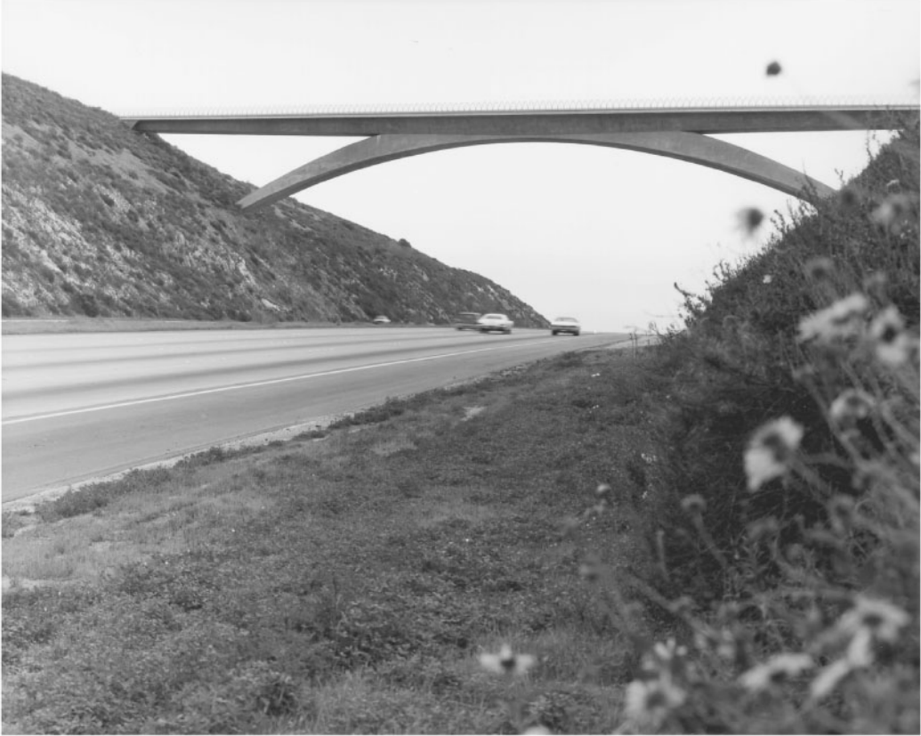
FIGURE 67.27 The Lilac Road arch gracefully frames the southern entrance to the fertile San Luis Rey Valley, of Southern California. It was built over Interstate Route 15 in San Diego County in 1978. The designer was Fred Michaels of the California Department of Transportation. (Courtesy of California Department of Transportation.)
