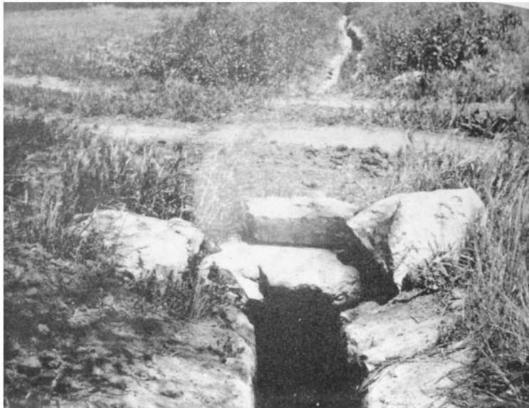
FIGURE 67.1 The aqueduct bridge at La Purisima Mission, Santa Barbara County, California, is an example of a primitive bridge, a short-span stone slab. Built in 1813, it is the oldest bridge in California. (Courtesy of California Department of Transportation.)
