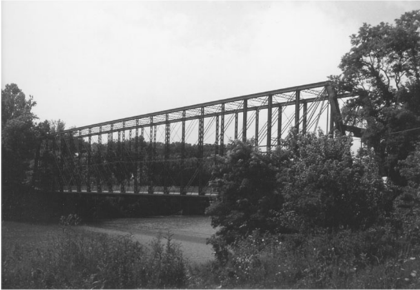
FIGURE 67.15 Laughery Creek Bridge, near Aurora, Indiana, was built by the Wrought Iron Bridge Company of Canton, Ohio, in 1878. Its 92-m span was unprecedented. This bridge appeared on the cover of the company’s catalog in 1893. (Courtesy of American Society of Civil Engineers.)
