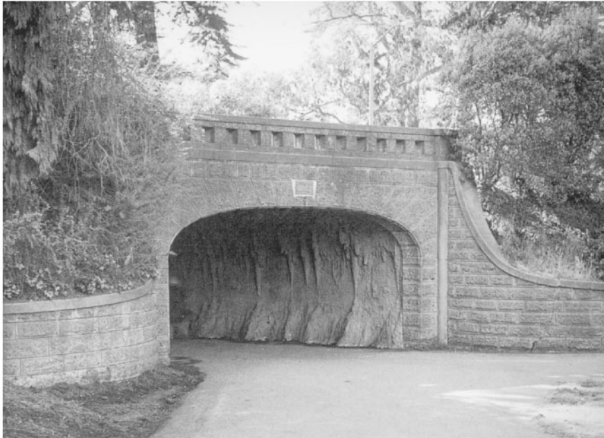
FIGURE 67.20 Alvord Lake Bridge is the first reinforced concrete bridge, built by Ernest Ransome, the developer of reinforced concrete, in 1888. This bridge is still in service carrying State Route 1 over Golden Gate Park in San Francisco. The fascia is hammered to resemble familiar stone arch work. The bridge is a National Historic Civil Engineering Landmark. (Courtesy of California Department of Transportation.)
