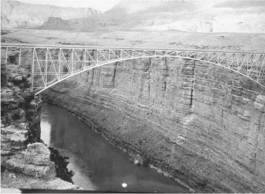
FIGURE 67.13 Navajo Bridge at Marble Canyon, near Lee's Ferry, Arizona, is the classic example of an arch sprung between canyon walls. This is also an example of a deck truss, an evolution for automobiles, beyond the through truss. When built, in 1929, it was the highest bridge in the world, 162.5 m, from deck to water. It was designed by Ralph Hoffman of the Arizona Highway Department. A parallel twin designed by Cannon Associates has since been constructed, in 1996. (Courtesy of American Society of Civil Engineers.)
