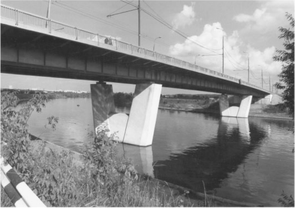
FIGURE 66.15 Moskva River Bridge in Krilatskoe.
