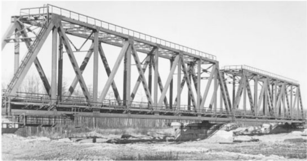
FIGURE 66.7 Typical through-truss bridge of 44 m span on the Baikal-Amour Railway Bridge Line.
