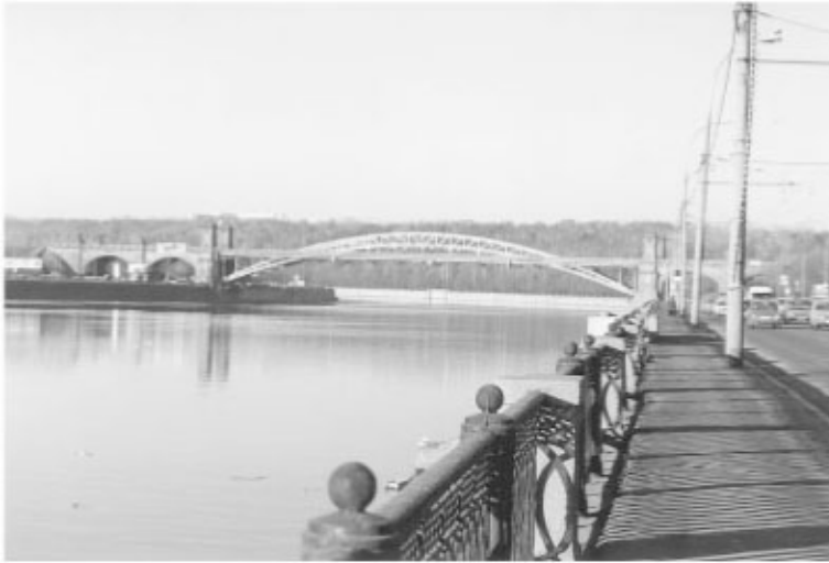
FIGURE 66.4 Steel depressed arch railway bridge over the Moskva River.
