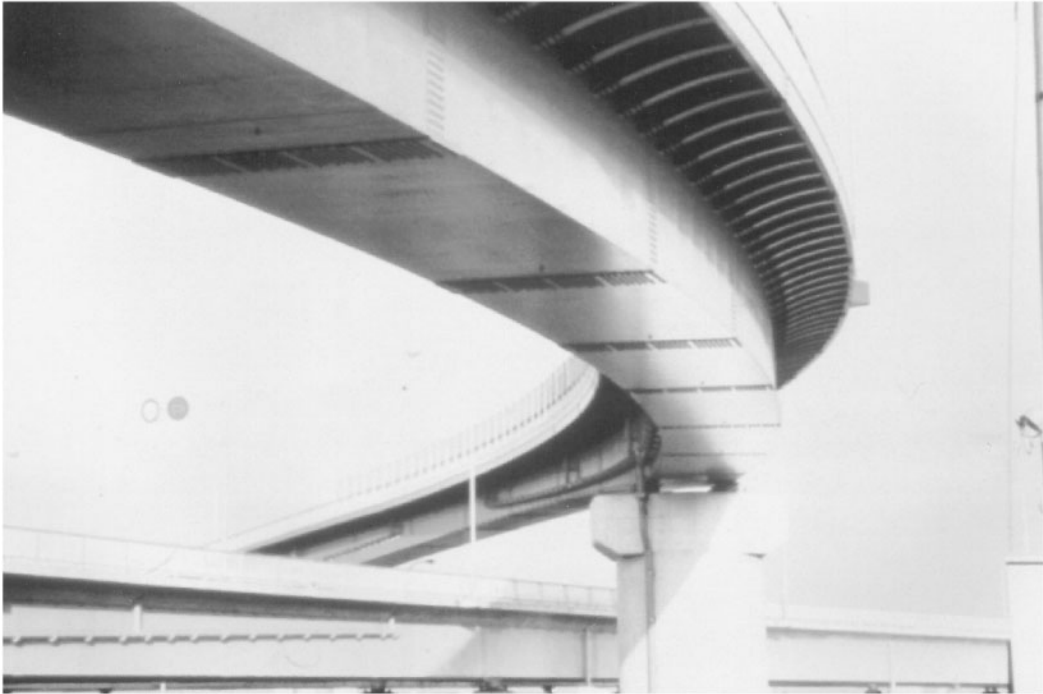
FIGURE 65.10 A curved tubular girder bridge in a metropolitan express highway.
