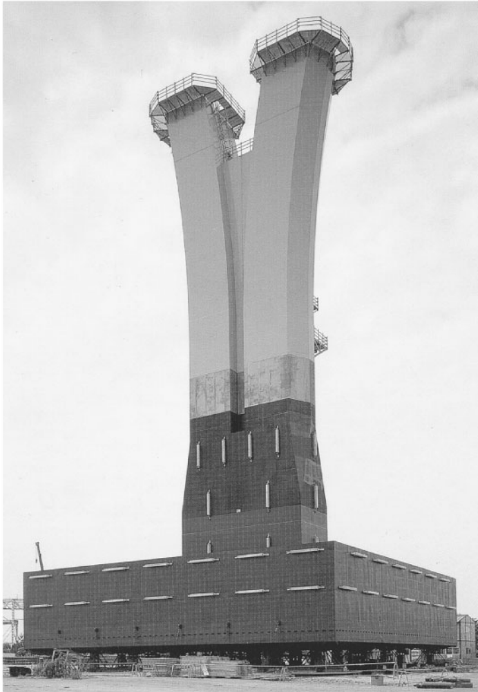
FIGURE 65.48 Steel pier with titanium-clad steel. (Courtesy of Nippon Steel.)
