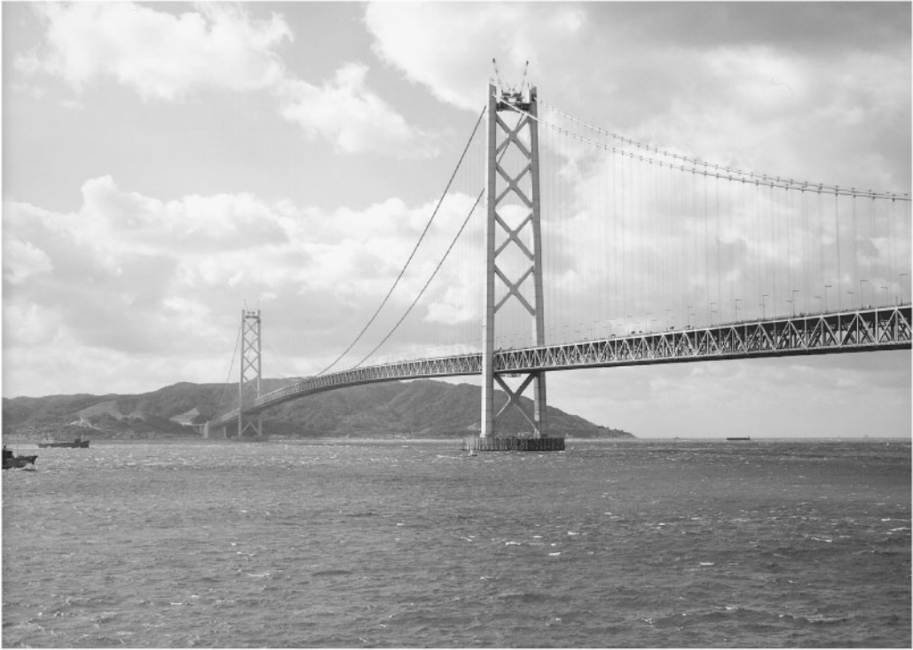
FIGURE 65.34 Akashi Kaikyo Bridge.
