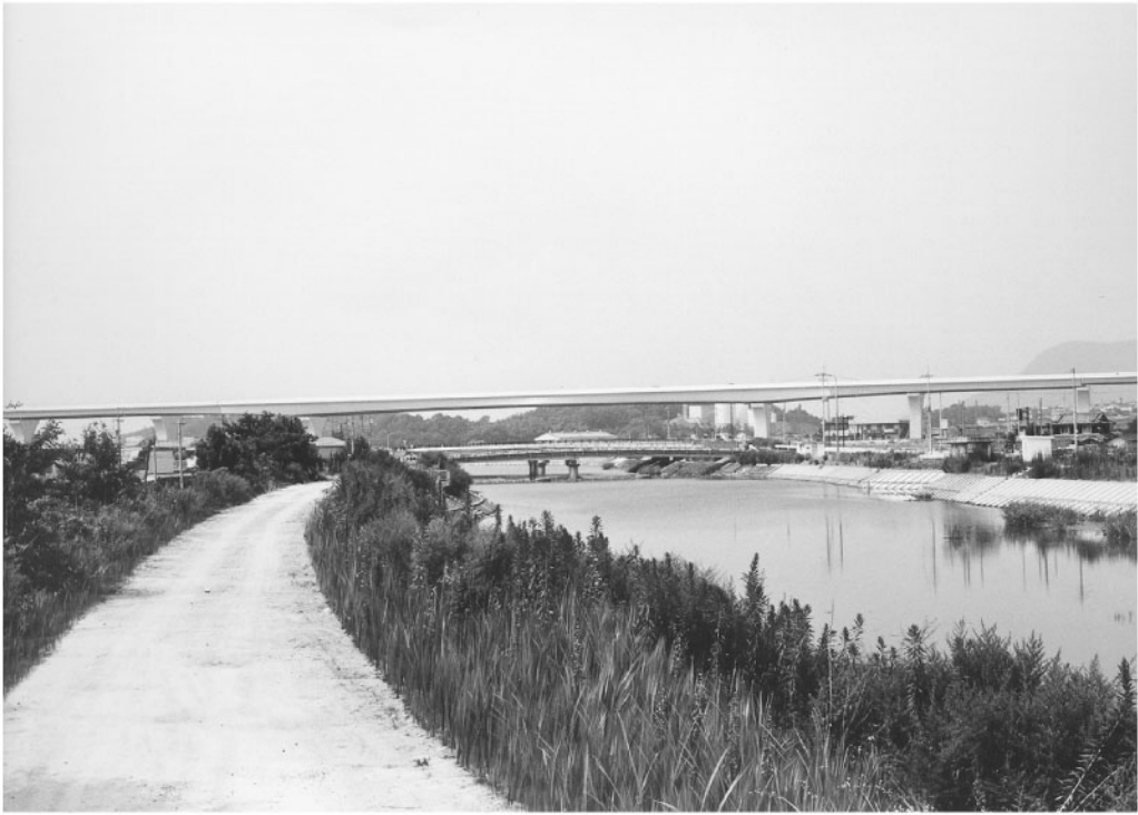
FIGURE 65.30 Shinkawa Bridge. (Courtesy of Japan Highway Public Corporation.)
