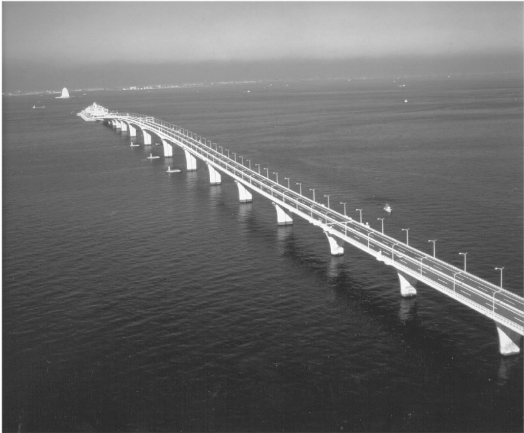
FIGURE 65.46 Steel bridges on Tokyo Wan Aqua-Line. (Courtesy of Trans-Tokyo Bay Highway Corporation.)
