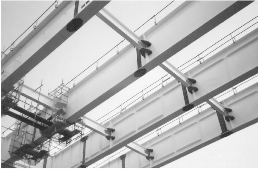
FIGURE 65.49 Plate I-girder with simple cross-beams.
