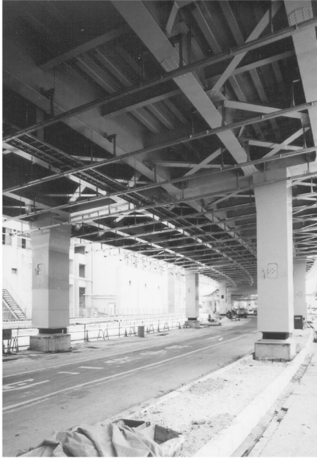
FIGURE 65.52 Rigid frame pier of Benten section. (Courtesy of Hanshin Expressway Public Corporation.)
