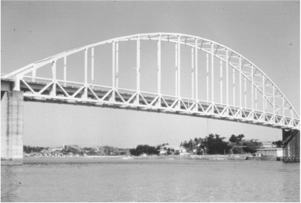
FIGURE 65.15 Ooyano Tsubasa Bridge.
