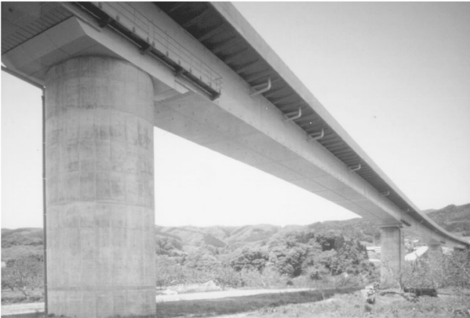
FIGURE 65.31 Kitachikuma Bridge. (Courtesy of Japan Highway Public Corporation.)
