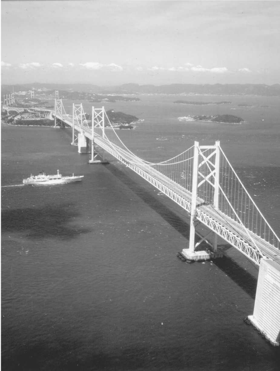
FIGURE 65.39 Kita-Bisan Seto and Minami-Bisan Seto Bridges.
