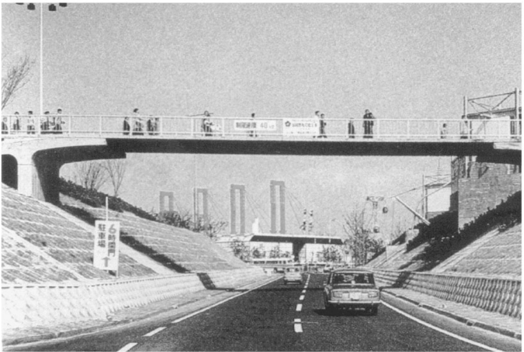
FIGURE 65.23 International Expo No. 9 Bridge.
