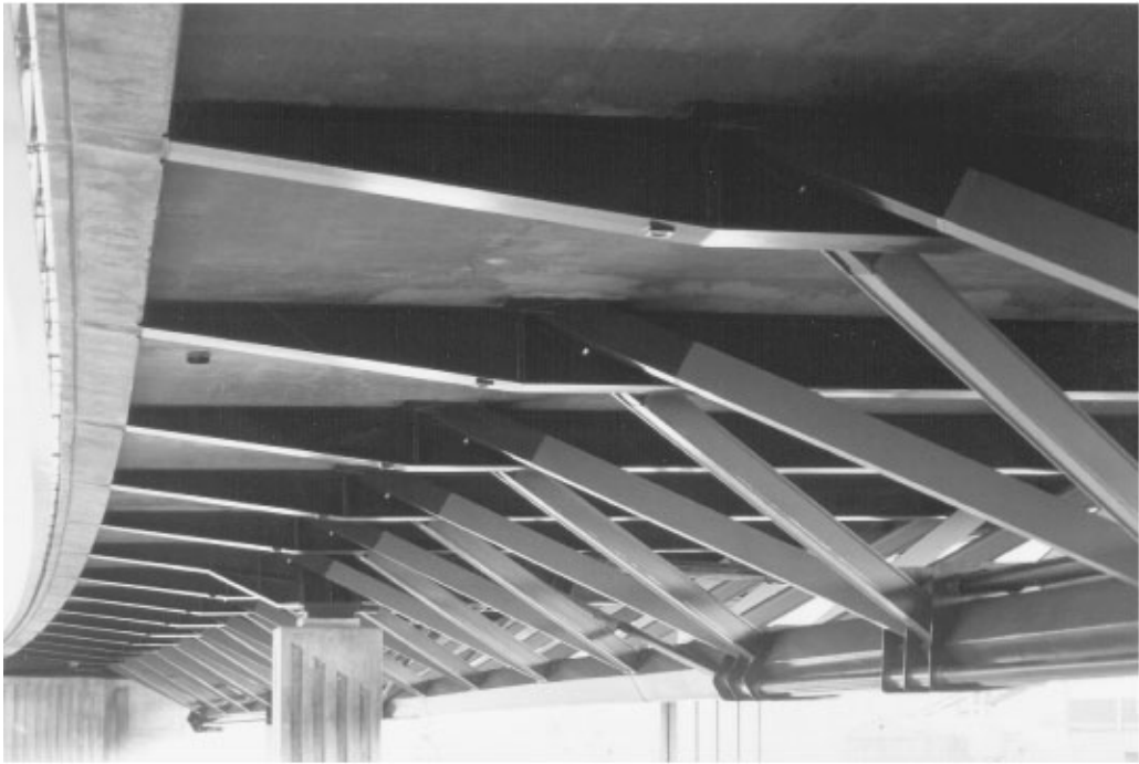
FIGURE 64.10 Roize Bridge. (Courtesy of Jean Muller International.)
