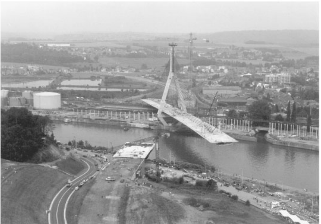
FIGURE 64.17 Ben Ahin Bridge during rotation. (Courtesy of Photo Studio 9 for Greisch.)
