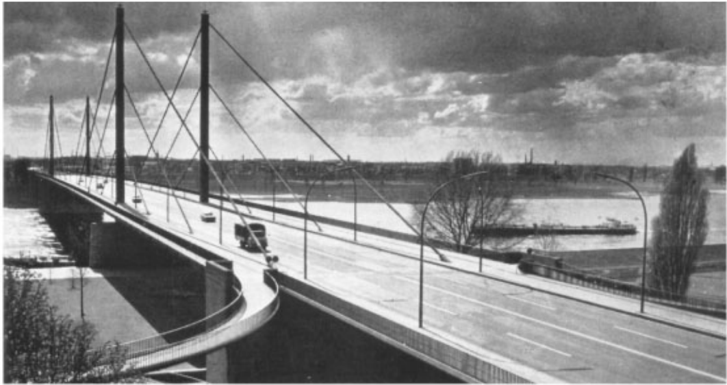
FIGURE 64.26 Theodor Heuss Bridge. (Source: Beyer, E., Bruckenbau, Beton Verlag, 1971. With permission.)
