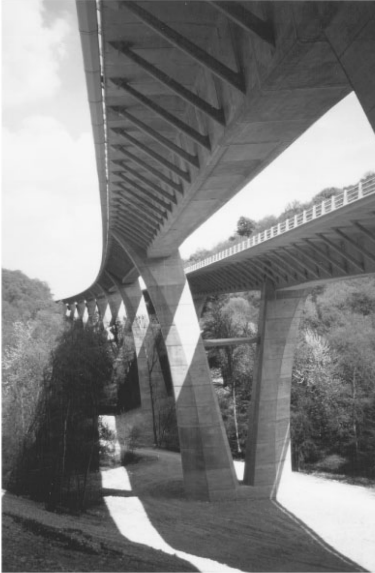
FIGURE 64.39 Rogerville Viaduct. (Courtesy of Jean Muller International.)
