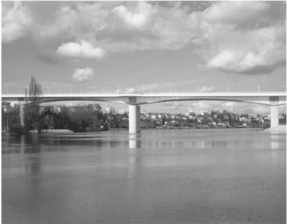
FIGURE 64.20 Dole Bridge. (Courtesy of Campenon Bernard.)
