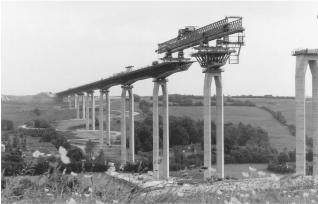
FIGURE 64.19 Boulonnais Bridges — pier transparency. (Courtesy of Jean Muller International.)
