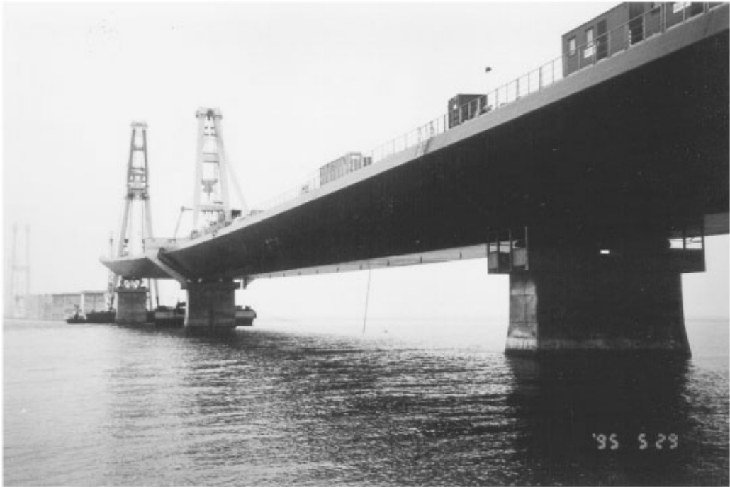
FIGURE 64.35 Great Belt Bridges — 193-m-long approach span. (Courtesy of Cowi Consult.)
