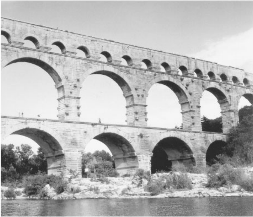
FIGURE 64.1 Gard Bridge over the River Gardon. (Source: Leonhardt, F, Ponts/Puentes — 1986 Presses Polytechniques Romandes. With permission.)
