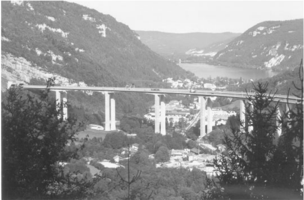
FIGURE 64.21 Nantua Viaduct. (Courtesy of Campenon Bernard.)
