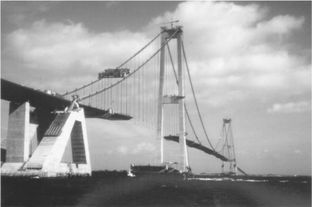
FIGURE 64.8 Storebælt Bridge. (Courtesy of Cowi Consult.)
