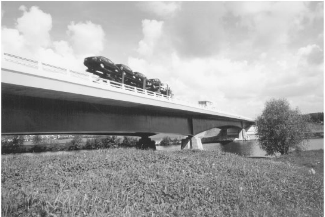
FIGURE 64.9 Oise Bridge. (Courtesy of Fred Boucher, SANEF.)
