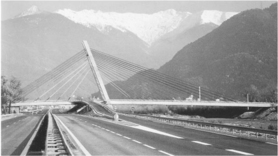
FIGURE 64.15 The Gilly Bridge. (Courtesy of Razel.)
