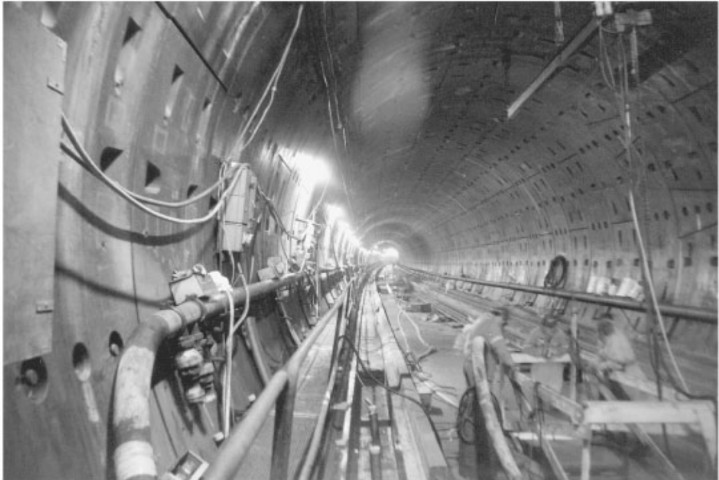
FIGURE 64.34 Great Belt Bridges — the railway tunnel. (Courtesy of Jean Muller International.)
