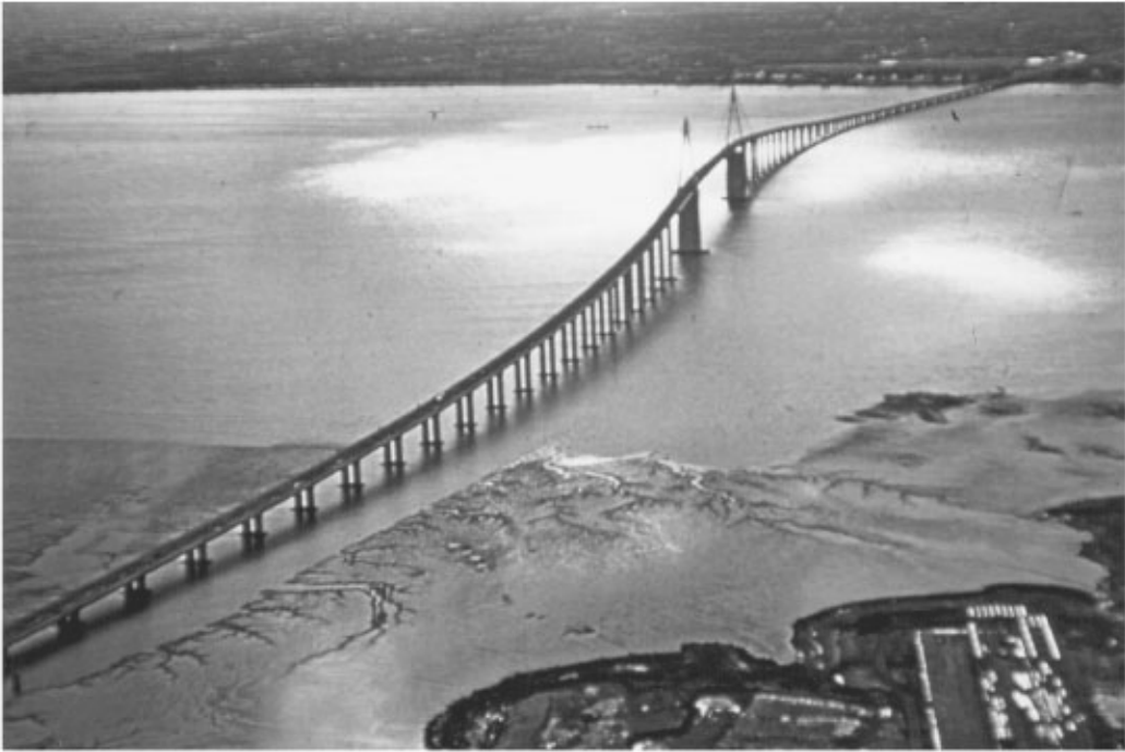
FIGURE 64.27 Saint Nazaire Bridge. (Courtesy of Jean Muller International.)
