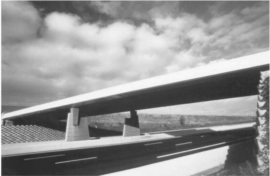
FIGURE 64.12 A1 highway overpasses. (Courtesy of J. P. Houdry, Egis Group.)
