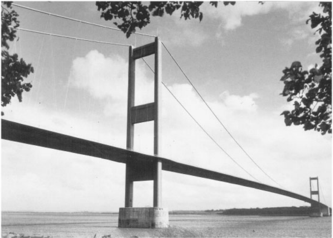
FIGURE 64.6 First Severn Bridge. ( Source: Leonhardt, F, Ponts/Puentes — 1986 Presses Polytechniques Romandes. With permission.)
