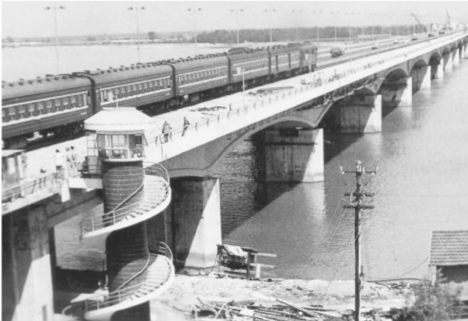
FIGURE 63.7 Second Qiantang River Bridge.
