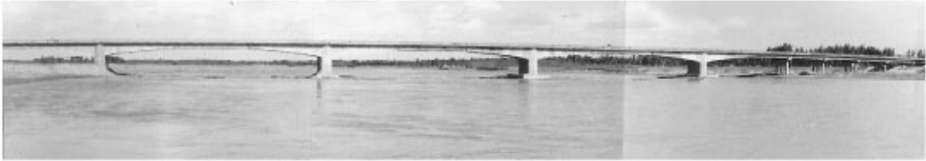
FIGURE 63.15 Qingtongxia Yellow River Highway Bridge.
