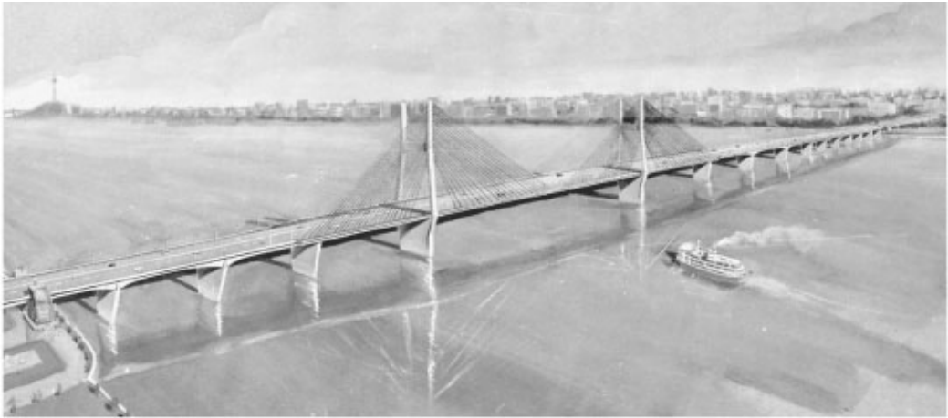
FIGURE 63.26 Wuhan Yangtze River Highway Bridge.
