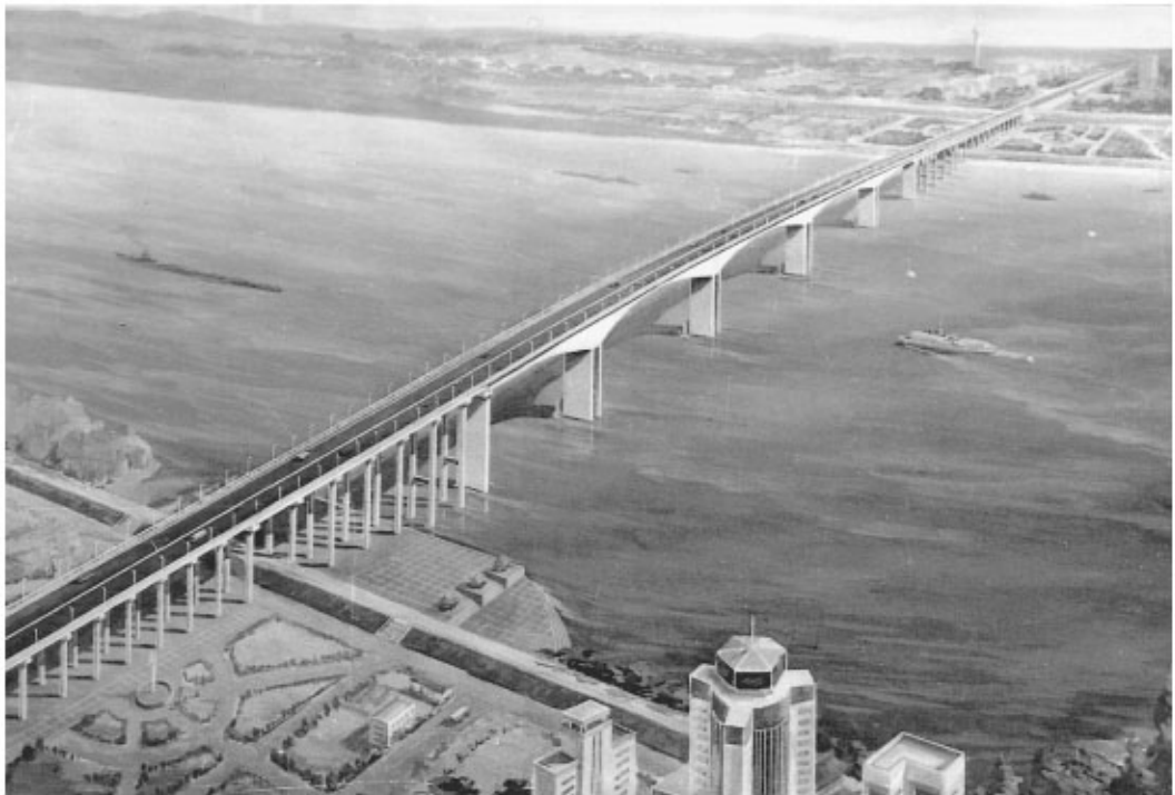
FIGURE 63.19 Huangshi Yangtze River Bridge.
