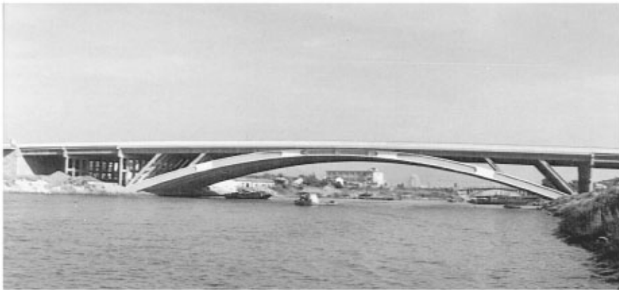
FIGURE 63.12 Jinkui Grand Canal Bridge.
