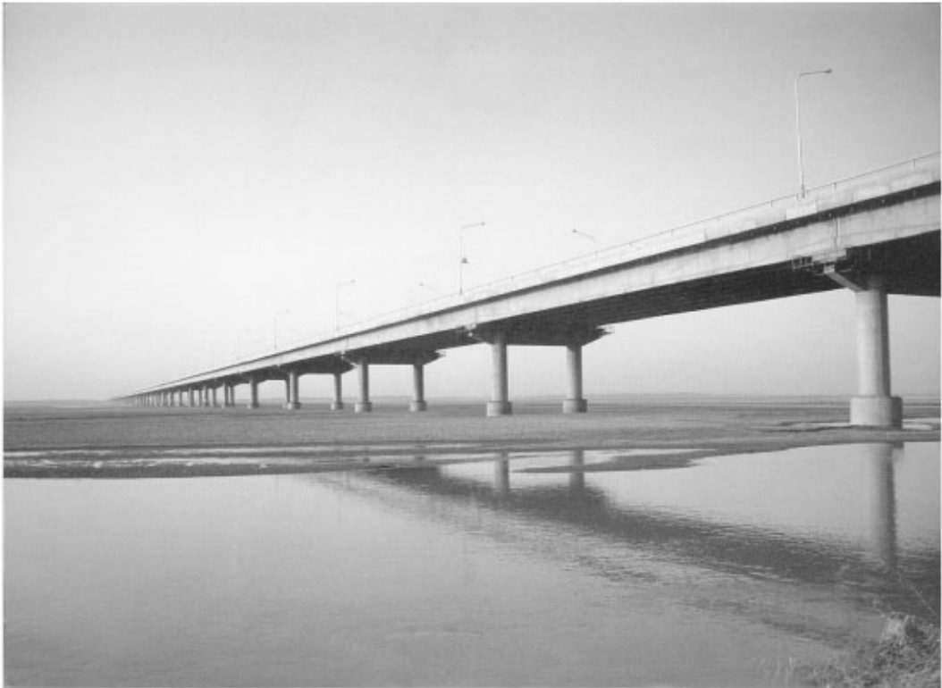
FIGURE 63.4 Kaifeng Yellow River Bridge.
