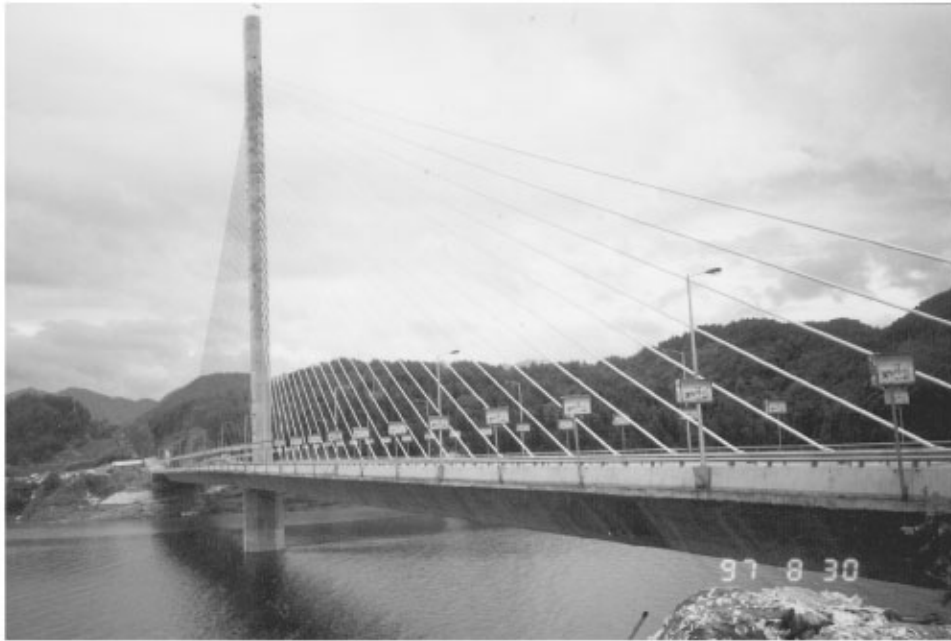
FIGURE 63.27 Huangshan Taiping Lake Bridge.
