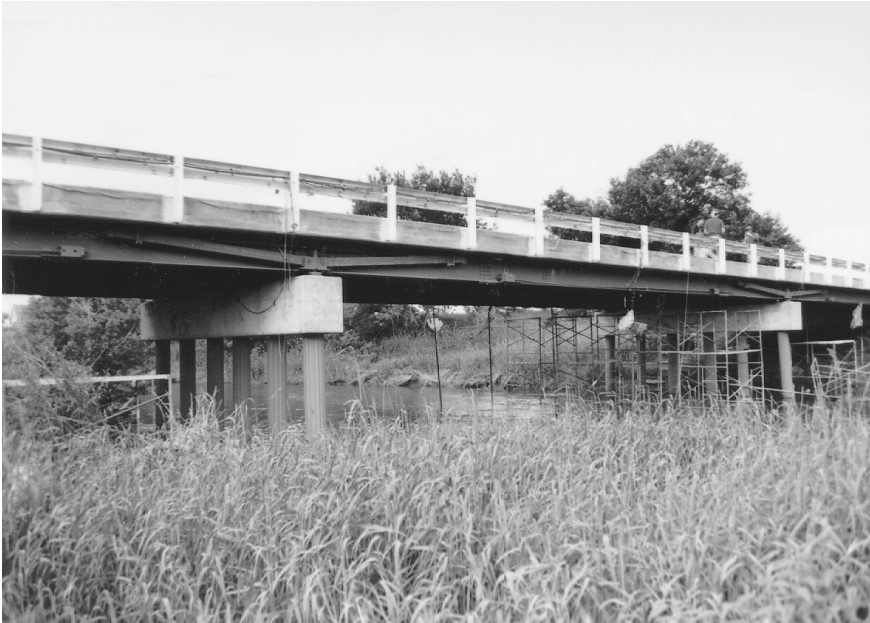
FIGURE 50.26 Photograph of three-span continuous bridge strengthened with post-tensioning and superimposed trusses.
