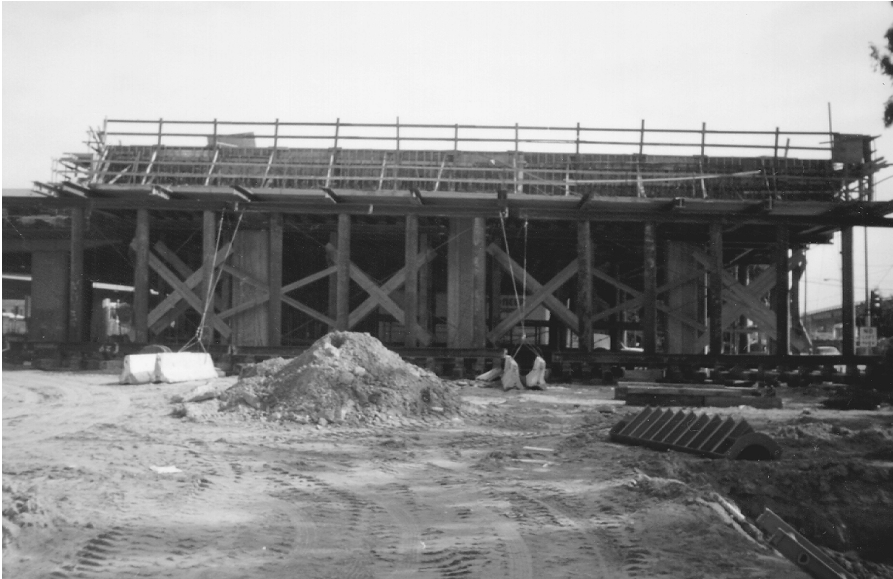
FIGURE 48.10 FW system for cast-in-place concrete bridge.
