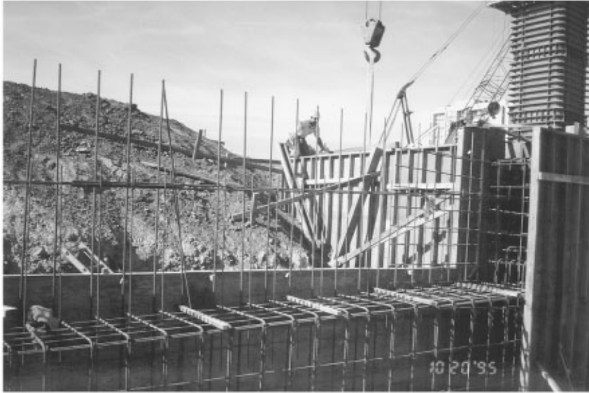
FIGURE 48.3 Wingwall and abutment construction.
