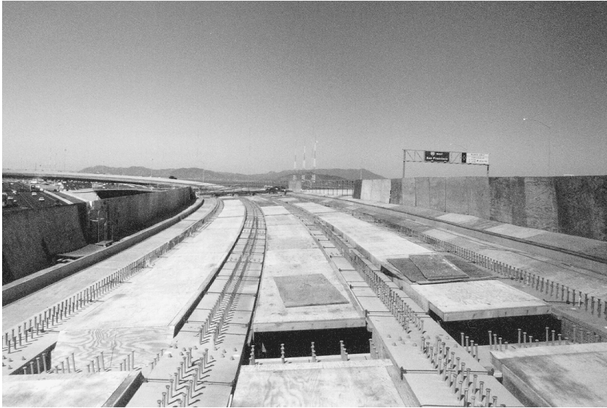
FIGURE 48.11 Temporary deck form for steel bridge.
