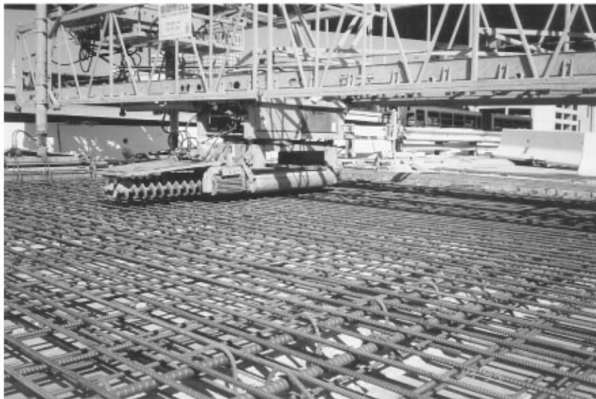
FIGURE 48.5 Bridge deck reinforcement with bidwell finishing machine.
