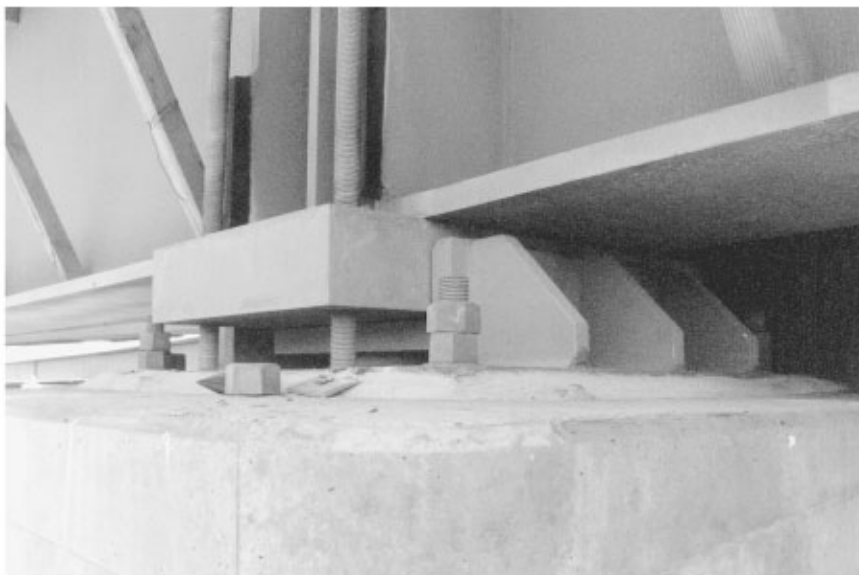
FIGURE 48.8 Bearing assembly of steel plate girder.
