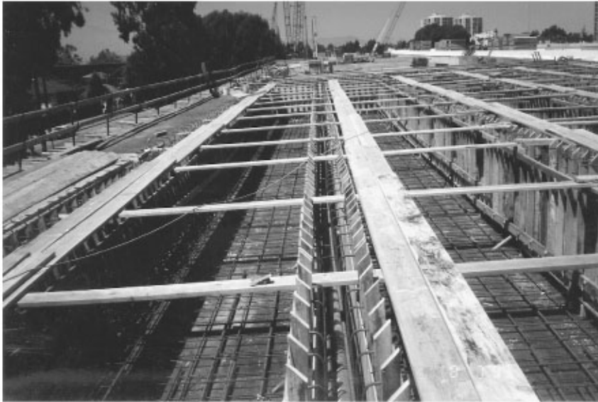
FIGURE 48.4 Bridge stem and soffit forms for concrete box girder.
