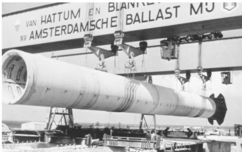
FIGURE 47.7 Prestressed concrete cylinder pile for Oosterschelde Bridge, the Netherlands.
