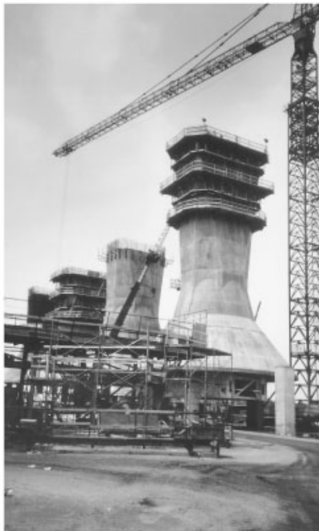
FIGURE 47.26 Prefabricated pier shaft and icebreaker, Prince Edward Island Bridge, Canada.
