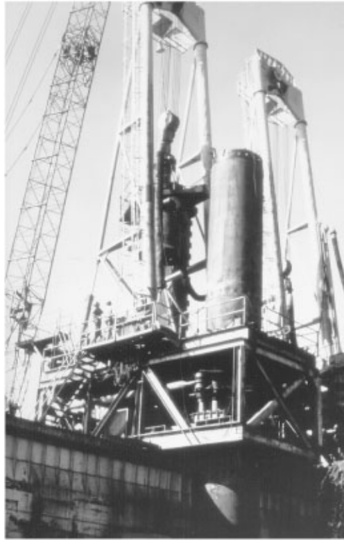
FIGURE 47.3 Steel tubular pile being installed from jack-up barge. Socket will be drilled into rock and entire pile filled with tremie concrete.
