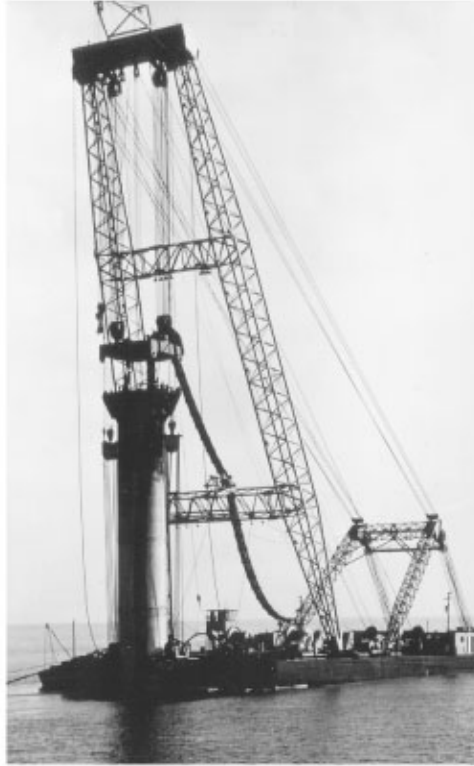
FIGURE 47.8 Installing concrete cylinder pile by internal excavation, jetting, and pull-down force from barge.
