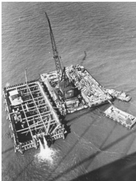
FIGURE 47.12 Dewatering the cofferdam for the main tower pier, Second Delaware Memorial Bridge.
