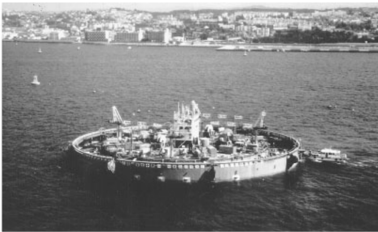
FIGURE 47.20 Akashi Strait Suspension Bridge is founded on steel box caissons filled with tremie concrete.
