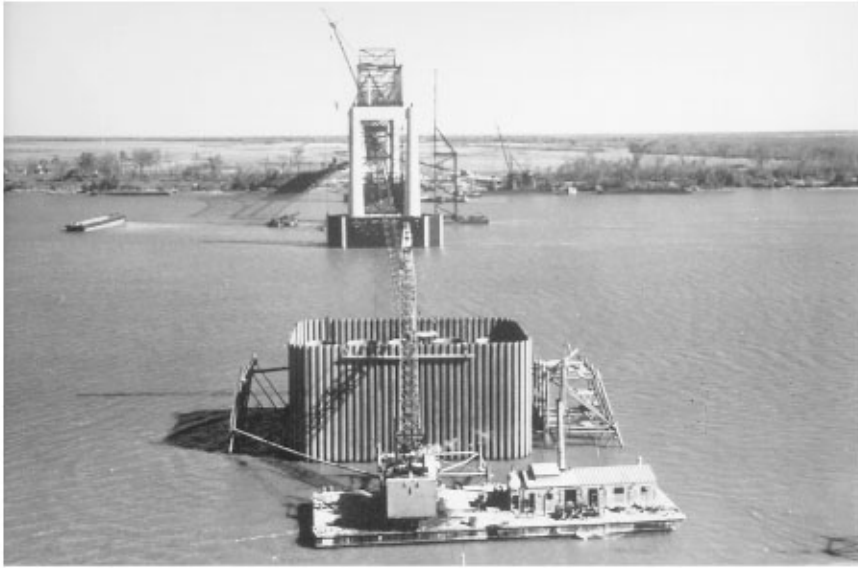
FIGURE 47.15 Open-caisson positioned within steel jackets on “pens.”
