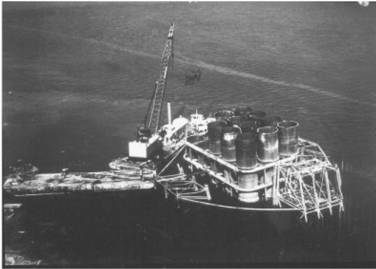
FIGURE 47.16 Open caisson for Sunshine Bridge across the Mississippi River. This caisson tipped during removal of false bottoms and is shown being righted by jacking against dolphins.
