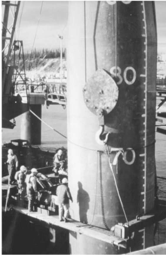
FIGURE 47.4 Large-diameter tubular steel pile being positioned.
