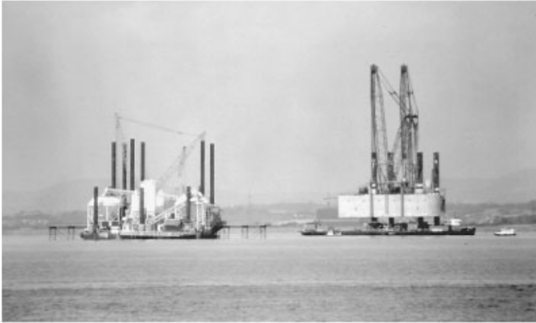
FIGURE 47.28 Installing precast concrete box caissons for Second Severn Crossing, Bristol, England. Extreme tidal range of 10 m and high tidal current imposed severe demands on installation procedures and equipment.
