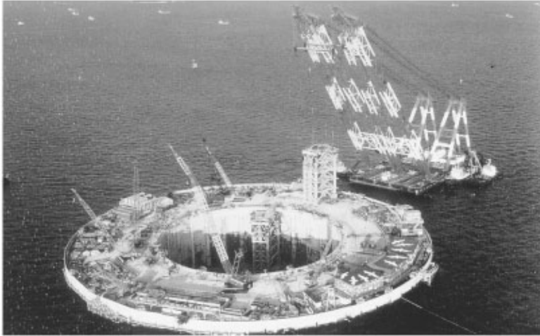
FIGURE 47.10 Slurry wall cofferdam for Kawasaki Island ventilation shaft, Trans-Tokyo Bay Tunnels and Bridge.
