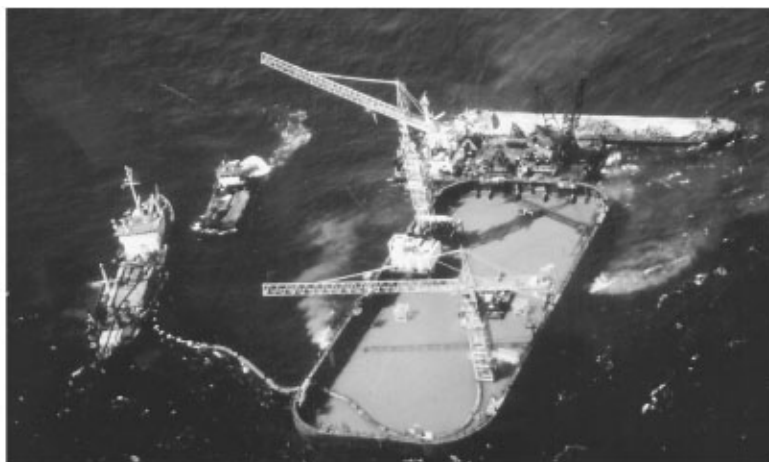
FIGURE 47.27 Prefabricated box caisson is floated into position, Great Belt Eastern Bridge, Denmark. Note temporary cofferdam above concrete caisson.
