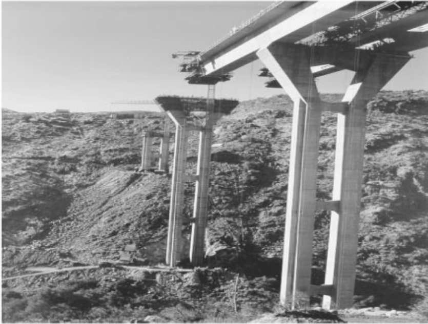
FIGURE 46.3 Pine Valley Creek Bridge — pier construction
