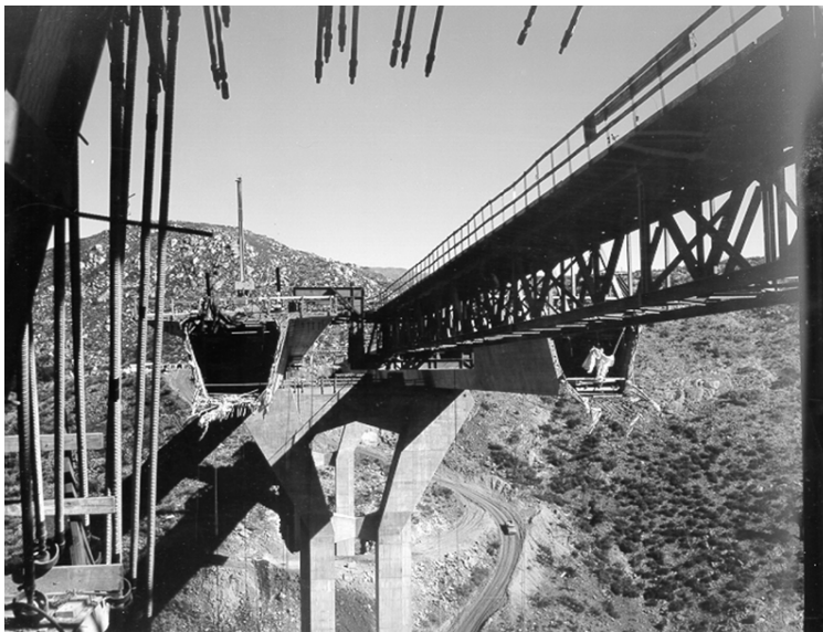
FIGURE 46.4 Pine Valley Creek Bridge — girder construction
