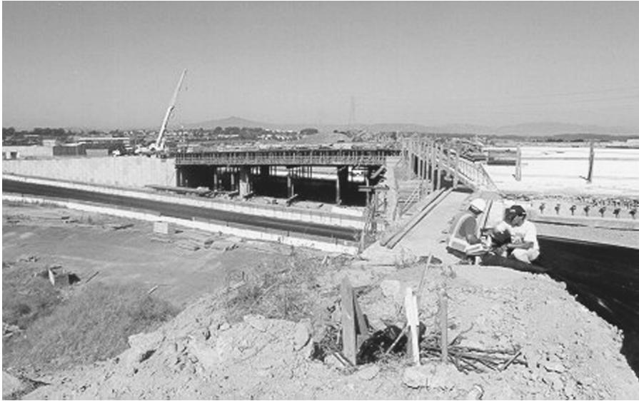
FIGURE 46.6 Falsework at I-80 HOV construction, Richmond, CA.
