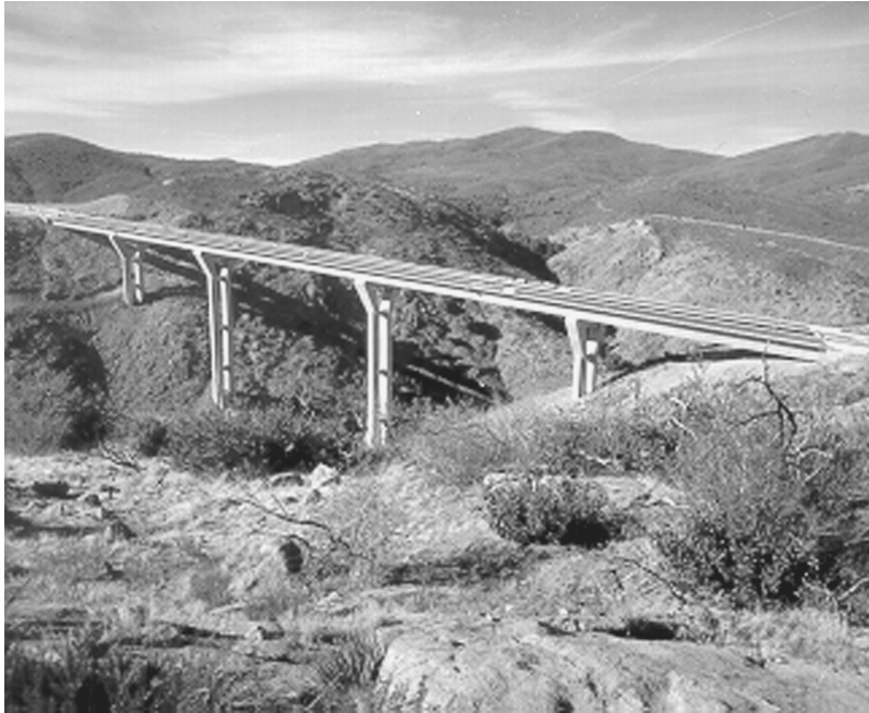
FIGURE 46.5 Pine Valley Creek Bridge — construction completion.
