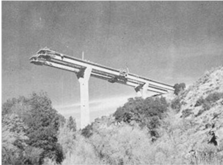
FIGURE 46.2 Pine Valley Creek Bridge — construction at Pier 4.
