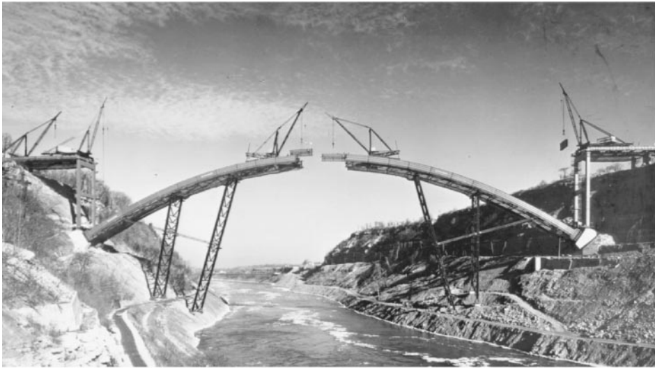
Figure 45.4 Lewiston-Queenston arch bridge, near Niagara Falls, New York, 1962. The longest fixed-arch span in the U.S. at 1000 ft (305 m); rise is 159 ft (48 m). Box arch-rib sections are typically about 3 \times 13\text{-}1/2 ft ( 0.9 \times 4.1 m) in cross-section and about 44\text{-}1/2 ft (13.6 m) long. Job was estimated using erection tiebacks (same as shown in Figure 45.3 ), but subsequent studies showed the long, sloping falsework bents to be more economical (even if less secure looking). Much permanent steelwork was used in the falsework bents. Derricks on approaches load steelwork onto material cars that travel up arch ribs. The 115-ton-capacity travelers are shown erecting the last full-length arch-rib sections, leaving only the short, closing crown sections to be erected. Canada is at left, the U.S. at right. (Courtesy of Bethlehem Steel Corporation.)
