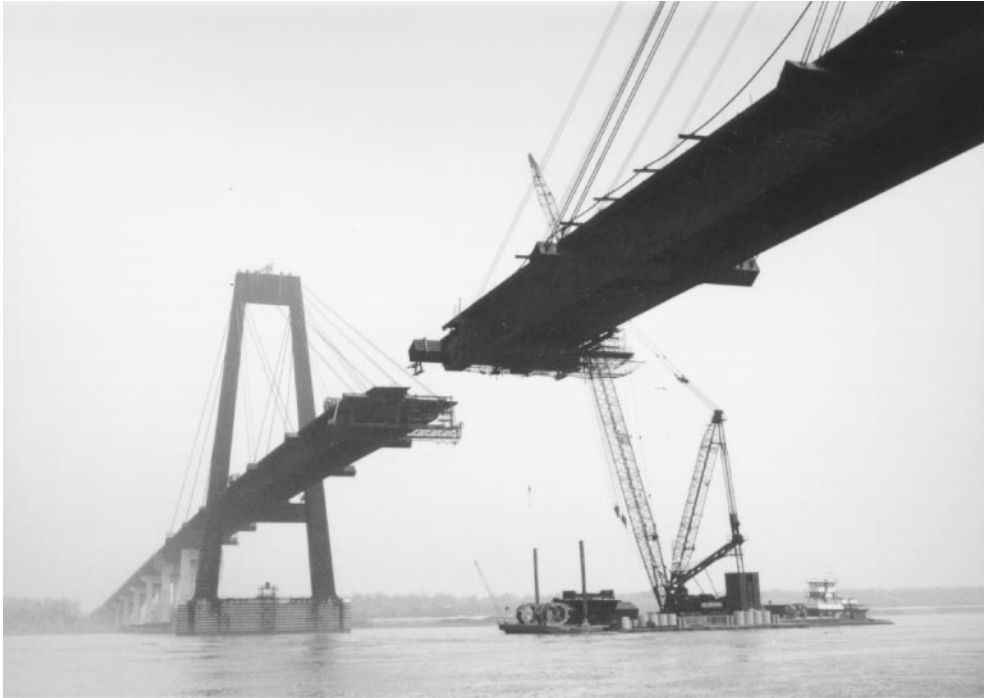
Figure 45.9 Cable-stayed orthotropic-steel-deck bridge over Mississippi River at Luling, La., 1982; view looking northeast. The main span is 1222 ft (372 m); the A-frame towers are 350 ft (107 m) high. A barge-mounted ringer derrick erected the main steelwork, using a 340 ft (104 m) boom with a 120 ft (37 m) jib to erect tower components weighing up to 183 tons, and using a shorter boom for deck components. Cable stays at the ends of projecting cross girders are permanent; others are temporary erection stays. Girder section 16-west of north portion of bridge, erected a few days previously, is projecting at left; companion girder section 16-east is on barge ready for erection (see Figure 45.10 ).
