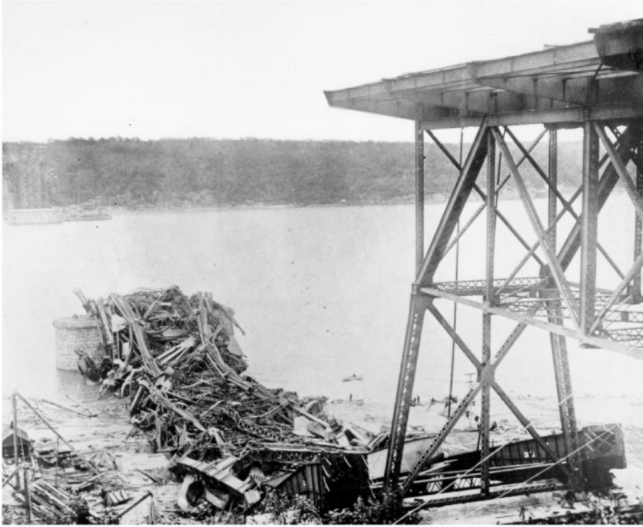
Figure 45.12 Wreckage of south anchor span of first Quebec railway cantilever bridge, 1907. View looking north from south shore a few days after collapse of 29 August 1907, the worst disaster in the history of bridge construction. About 20,000 tons of steelwork fell into the St. Lawrence River, and 75 workmen lost their lives.
