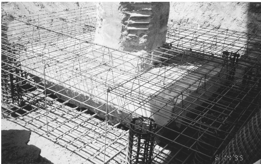
FIGURE 40.16 Typical footing and pile cap modification.
