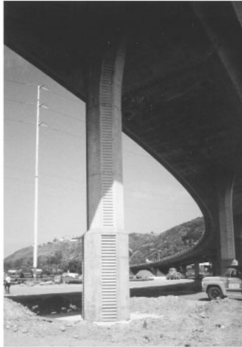
FIGURE 40.7 Concrete jacket column retrofit.
