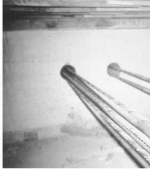
FIGURE 40.3 Hinge joint restrainer.
