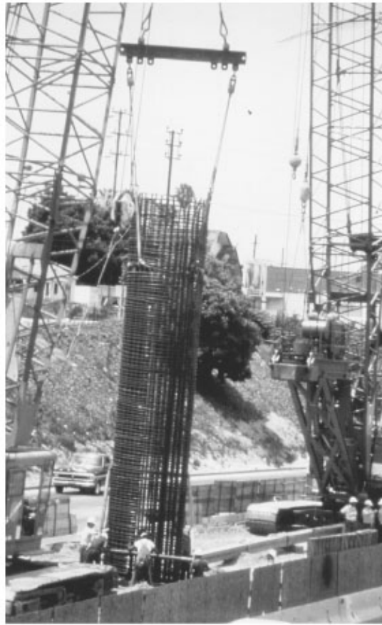
FIGURE 40.11 Column reinforcing steel cage.
