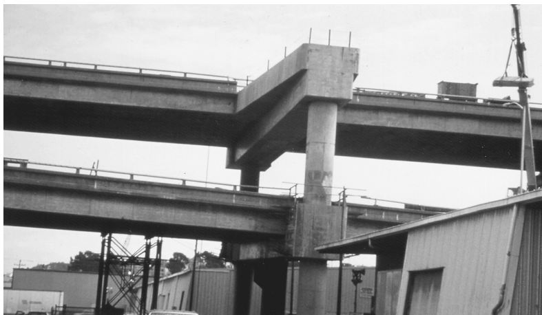
FIGURE 40.14 Completed retrofitted structures.
