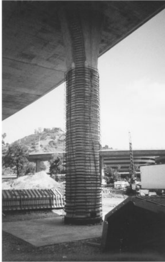
FIGURE 40.6 Reinforcement confinement retrofit.
