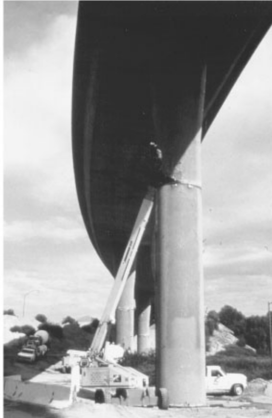
FIGURE 40.8 Steel jacket column retrofit.
