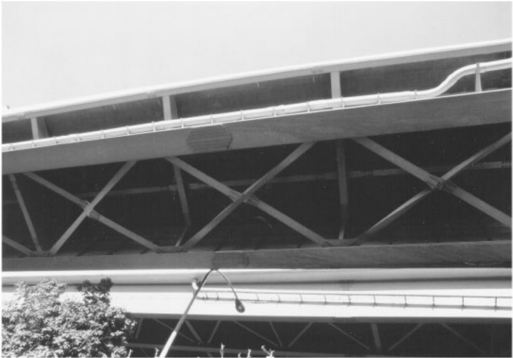
FIGURE 34.12 Buckling of braces near pier 209 of the Hanshin Expressway in the 1995 Hyogo-Ken Nanbu earthquake.
