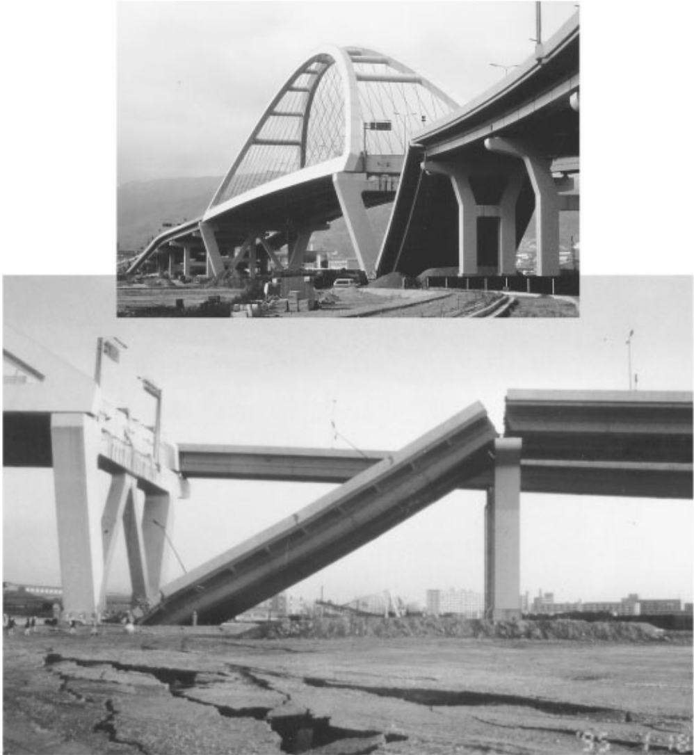
FIGURE 34.3 Nishinomiya-ko Bridge approach span collapse in the 1995 Hyogo-Ken Nanbu earthquake [Kobe Collection, EERC Library, University of California, Berkeley].
