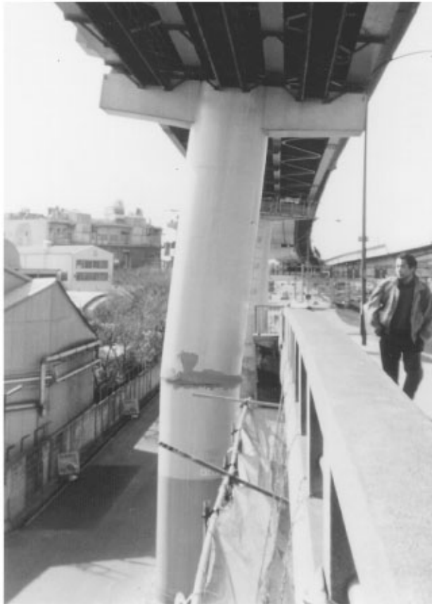
FIGURE 34.25 Local buckling of a circular cross-section column of the Hanshin Expressway in the 1995 Hyogo-Ken Nanbu earthquake.
