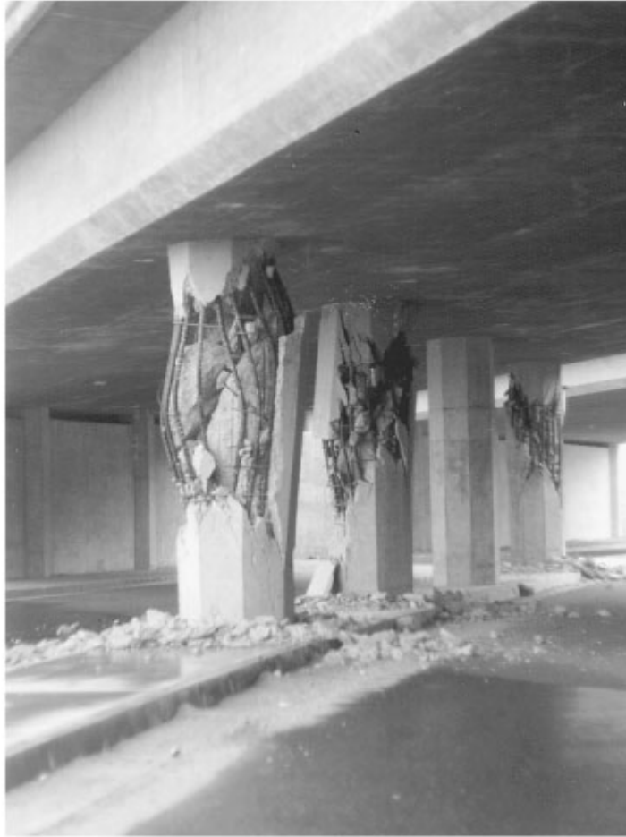
FIGURE 34.20 Failure of columns of the Route 5/210 interchange during the 1971 San Fernando earthquake.
