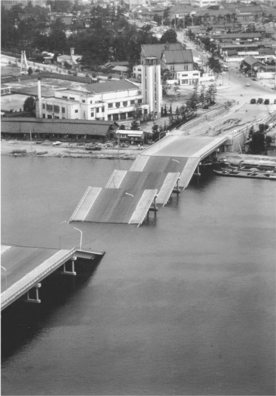
FIGURE 34.8 Showa Bridge collapse in 1964 Niigata earthquake.
