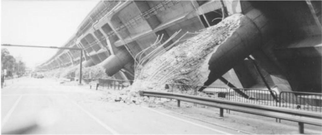
FIGURE 34.4 Higashi-Nada Viaduct collapse in the 1995 Hyogo-Ken Nanbu earthquake. (Source: EERI, The Hyogo-Ren Nambu Earthquake, January 17, 1995, Preliminary Reconnaissance Report, Feb. 1995.)
