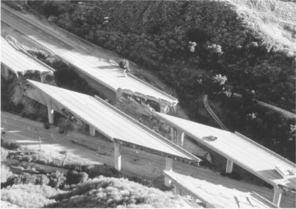
FIGURE 34.10 Gavin Canyon Undercrossing collapse in the 1994 Northridge earthquake.
