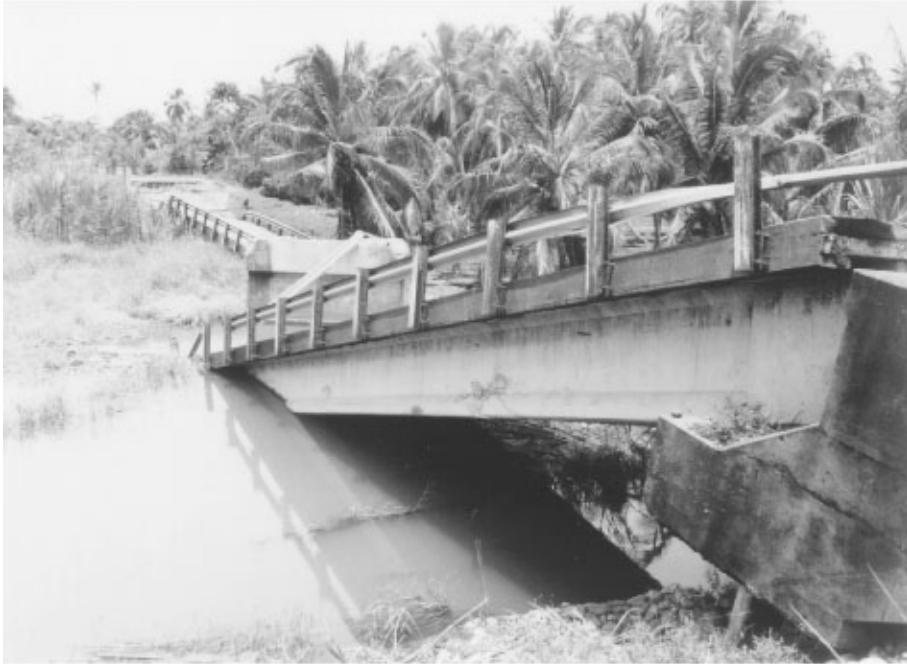
FIGURE 34.9 Rio Bananito Bridge collapse in the 1991 Costa Rica earthquake. (Source: EERI, Earthquake Spectra , Special Suppl. to Vol. 7, 1991.)
