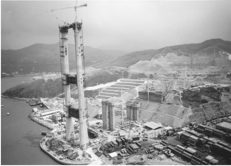
FIGURE 18.27 Tower erection for the Tsing Ma Bridge. (Courtesy of Mitsui Engineering & Shipbuilding Co., Ltd.)
