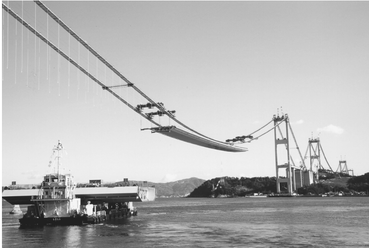
FIGURE 18.31 Block erection method on the Kurushima Kaikyo Bridge. (Courtesy of Honshu–Shikoku Bridge Authority.)
