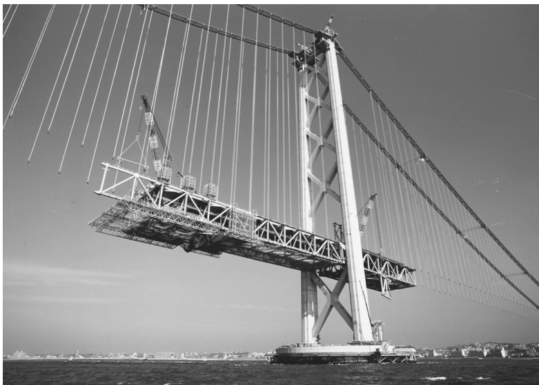
FIGURE 18.32 Cantilevering method in the Akashi Kaikyo Bridge. (Courtesy of Honshu–Shikoku Bridge Authority.)
