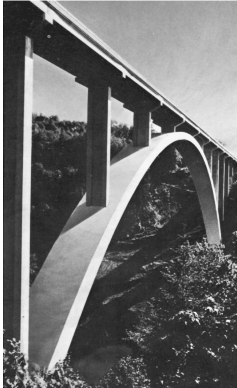
FIGURE 17.5 Cowlitz River concrete arch.
