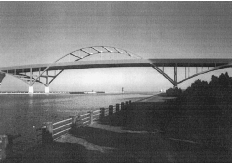
FIGURE 17.8 Milwaukee Harbor half-through arch.
