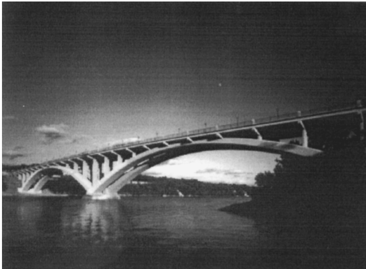
FIGURE 17.6 Two shallow concrete arch spans.
