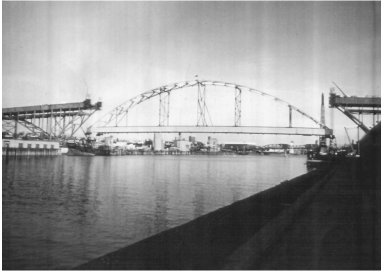
FIGURE 17.15 Fremont tied arch being lifted into place.
