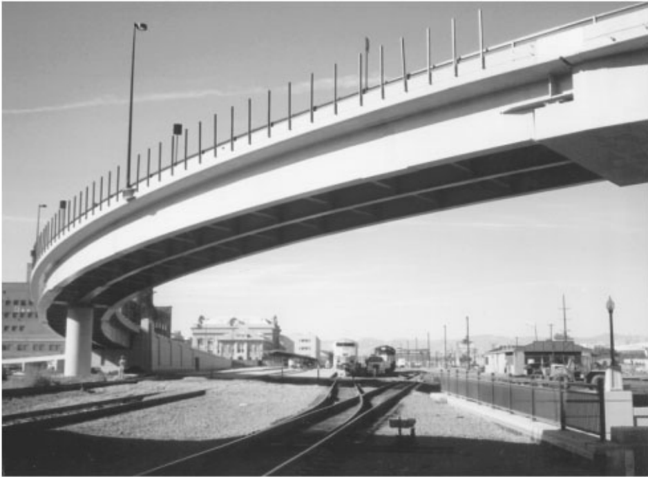
FIGURE 15.3 Curved I-girder bridge with integral bent cap.
