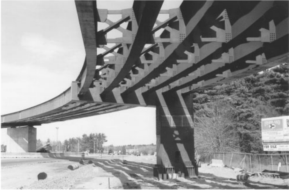
FIGURE 15.1 Curved I-girder bridge under construction — 20th St. HOV, Denver, Colorado.
