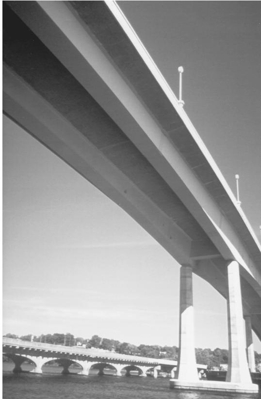
FIGURE 15.4 Twin box-girder bridge — U.S. Naval Academy Bridge, Annapolis, Maryland.
