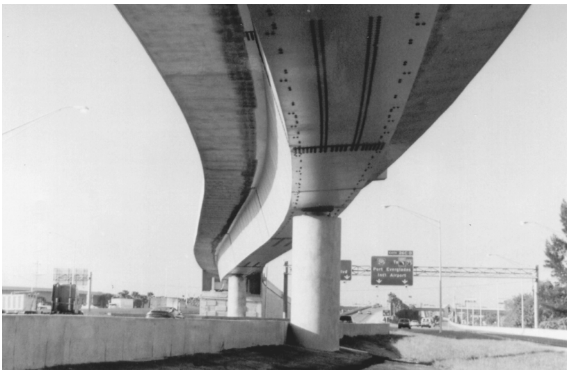
FIGURE 15.5 Single box girder bridge with integral bent cap — Ramp Y, I-95 Davies Blvd., Broward County, Florida.
