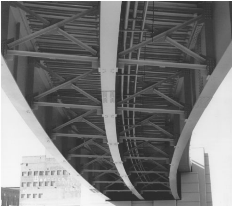
FIGURE 15.2 Bottom view of curved I-girder bridge.
