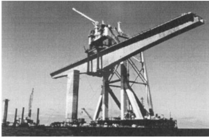
FIGURE 11.52 Confederation Bridge, Canada — floating crane.
