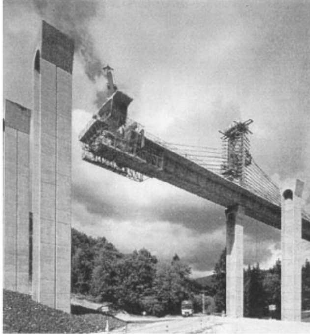
FIGURE 11.7 Fréburge Viaduct, France—erection with movable stay tower.
