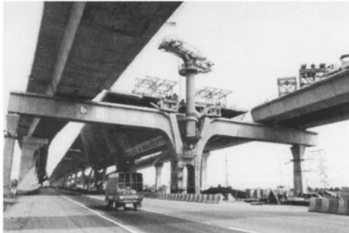
FIGURE 11.53 Bang Na–Bang Pli–Bang Pakong Expressway, Thailand — D6 segment erection.
