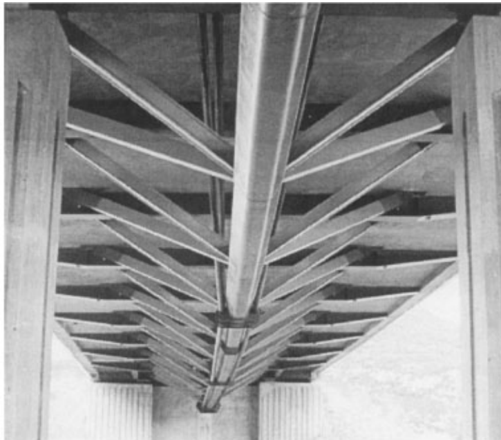
FIGURE 11.12 View of the Roize Bridge, France — space truss spans using tetrahedron modules.
