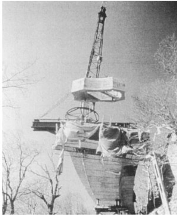
FIGURE 11.9 Linn Cove Viaduct — pier being constructed from the deck level.
