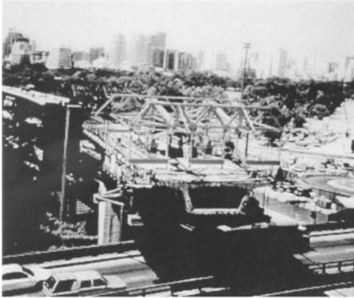
FIGURE 11.3 Construction of the Bangkok Transit System over Rama IV Flyover, Thailand.
