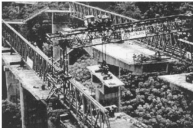
FIGURE 11.51 H-3 Windward Viaduct, Hawaii.
