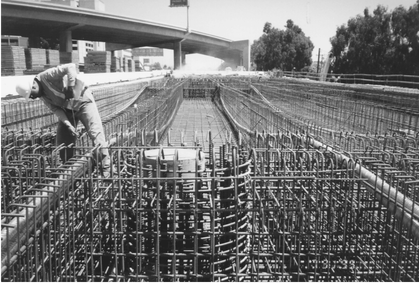
FIGURE 10.2 A post-tensioned box-girder bridge under construction.
