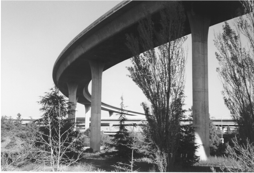
FIGURE 10.4 Prestressed box-girder bridge (I-280/110 Interchange, CA).
