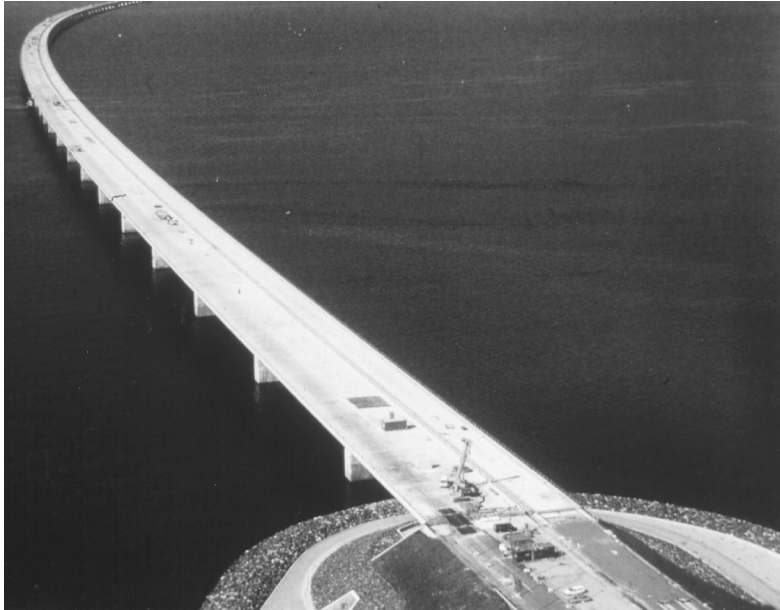
FIGURE 4.5 Storebælt West Bridge.
