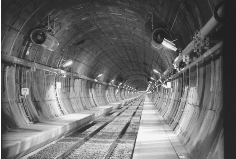
FIGURE 4.6 Storebælt East Tunnel.
