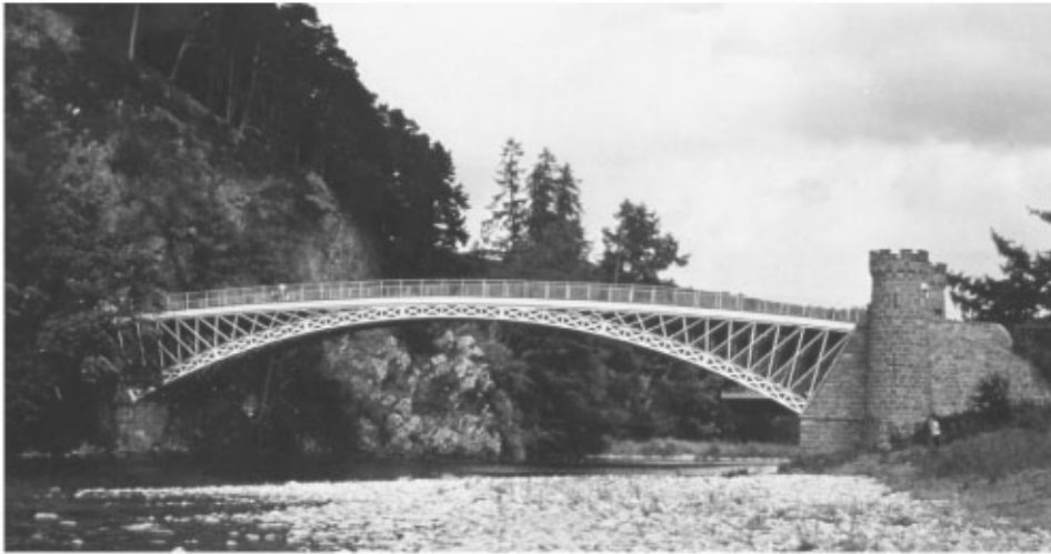
FIGURE 3.1 Thomas Telford's Craigellachie Bridge.
