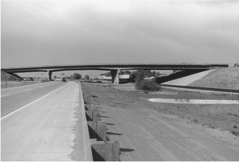
FIGURE 3.10 Buckley Road over I-76.
