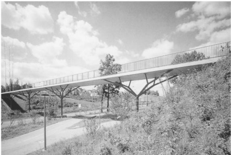
FIGURE 3.4 One of Jorg Schlaich's footbridges.
