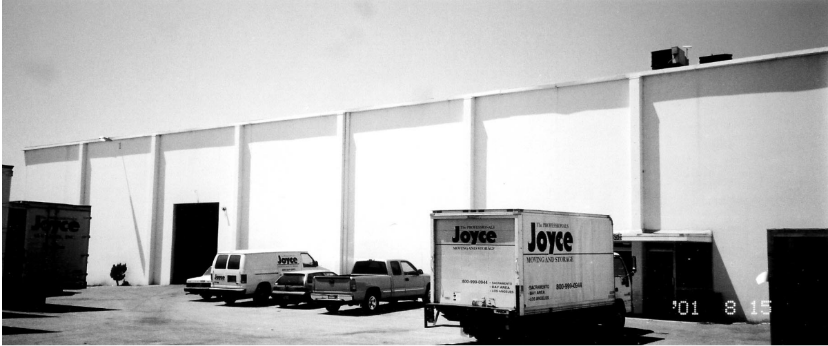
Fig. 2.1 View of tilt-up wall building looking west
