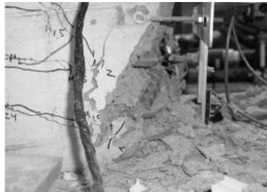
Fig. 13—Buckling of reinforcement in Unit 3.
