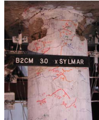
b) West Column –South View
