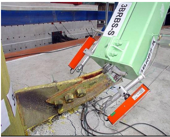
Figure 17. Buckling of the gusset at the brace to column joint after Phase-1 tests.
