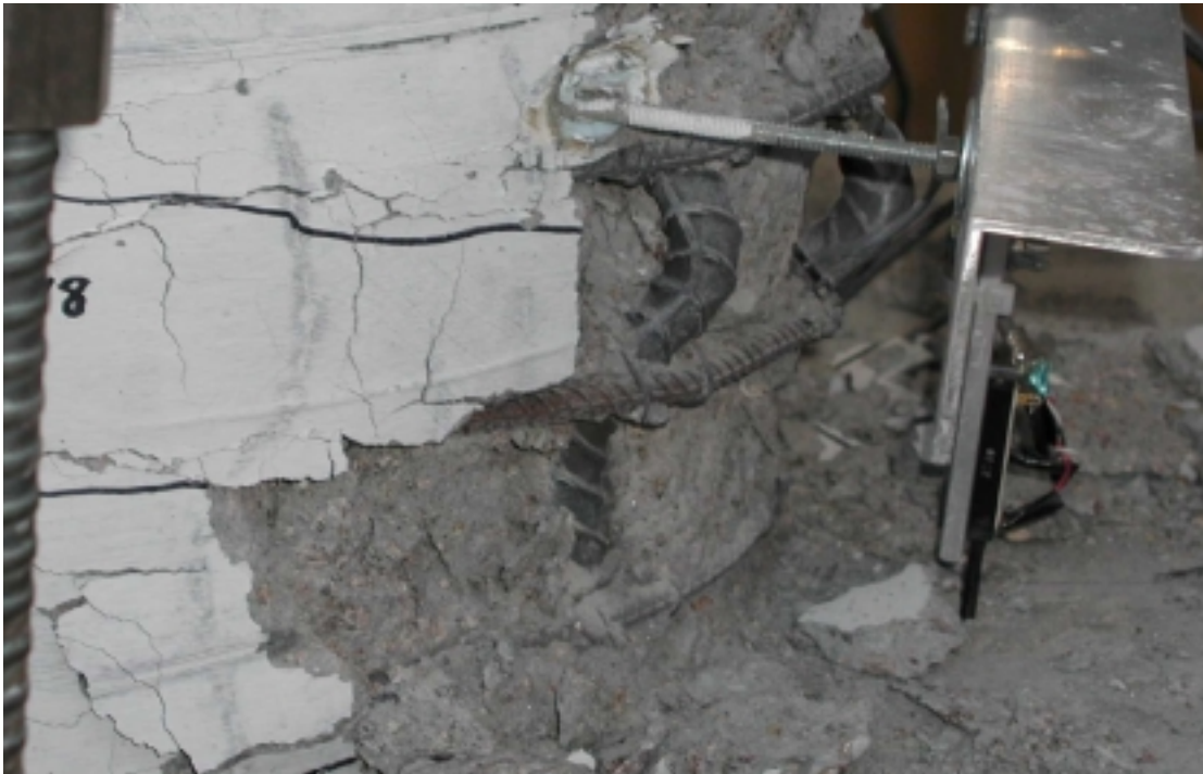
Figure 11.16 North Side of Specimen at Failure
