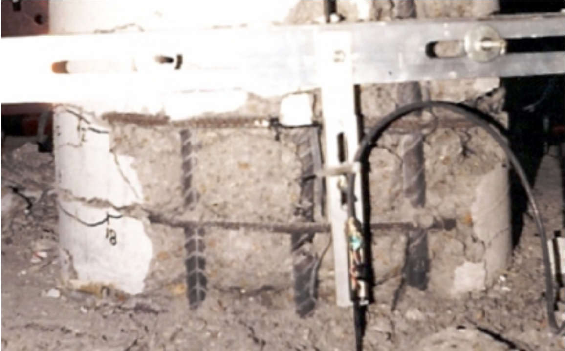
Figure 9.13 Rupture of Reinforcement North Side of Specimen at Ductility 7
