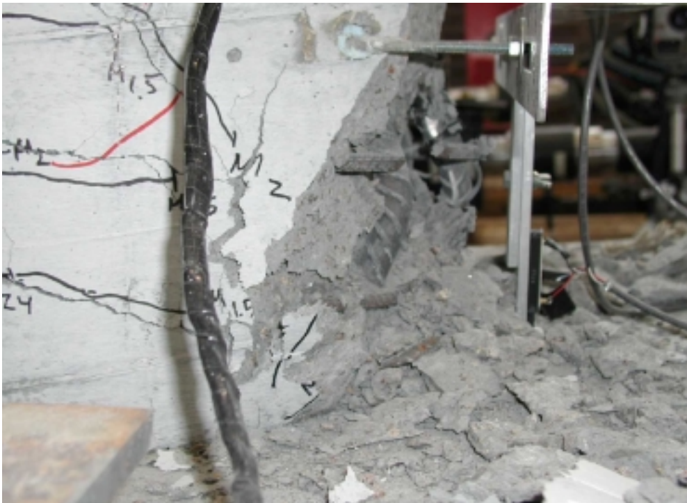
Figure 10.17 South Side of Specimen at Failure
