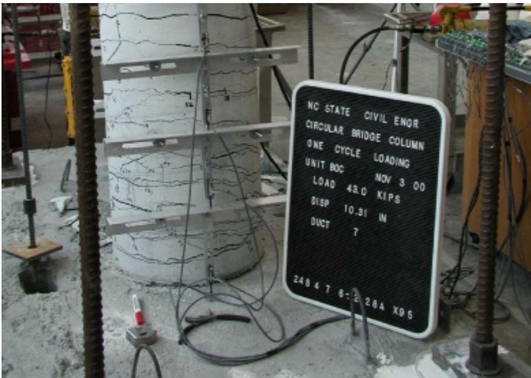
Figure 10.13 South Side of Specimen at Ductility 7
