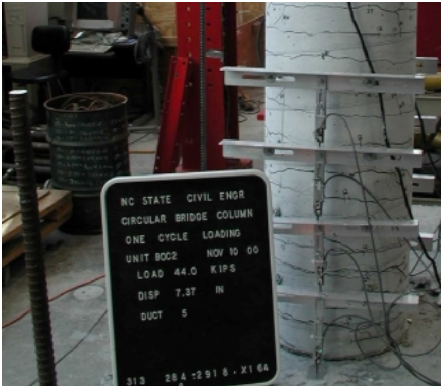
Figure 11.9 North Side of Specimen at Ductility 5
