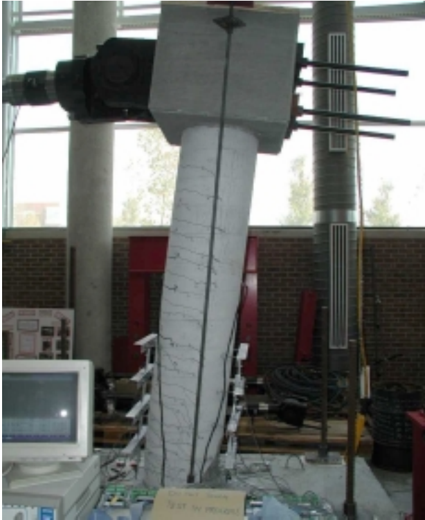
Figure 10.14 West Side of Specimen at Ductility 7
