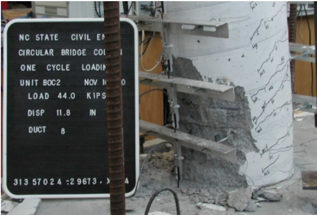
Figure 11.12 South Side of Specimen at Ductility 8
