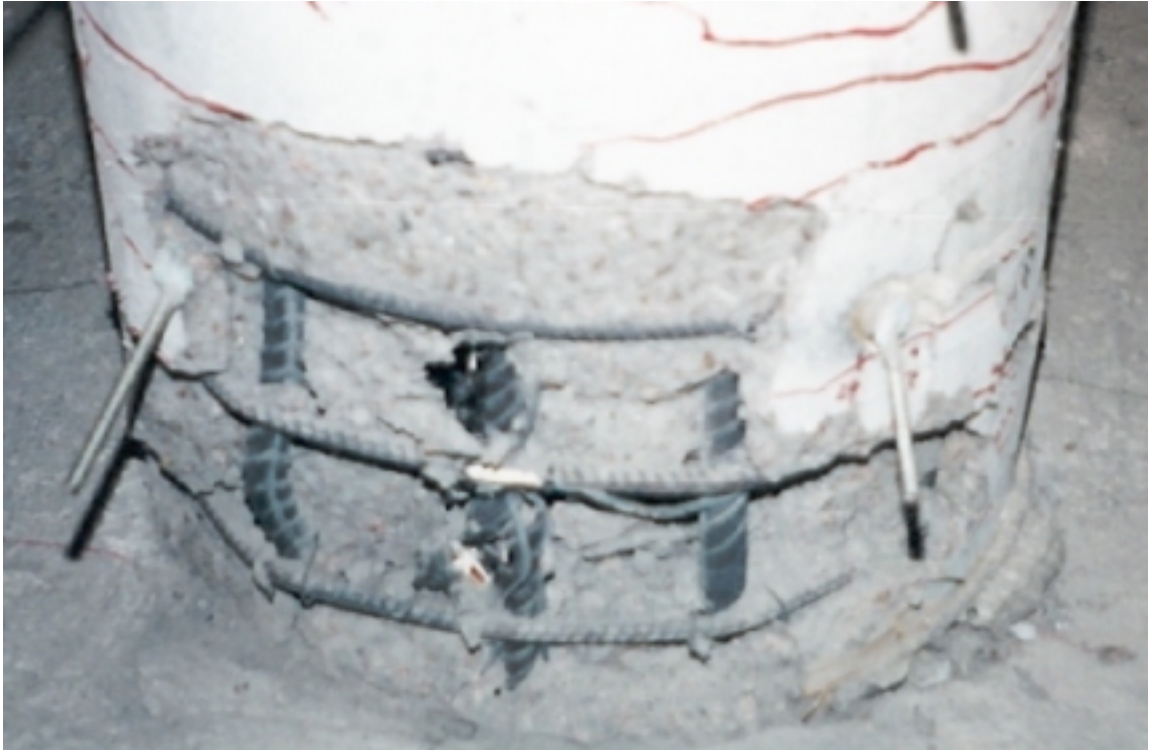
Figure 8.10 South Side of Specimen after Test
