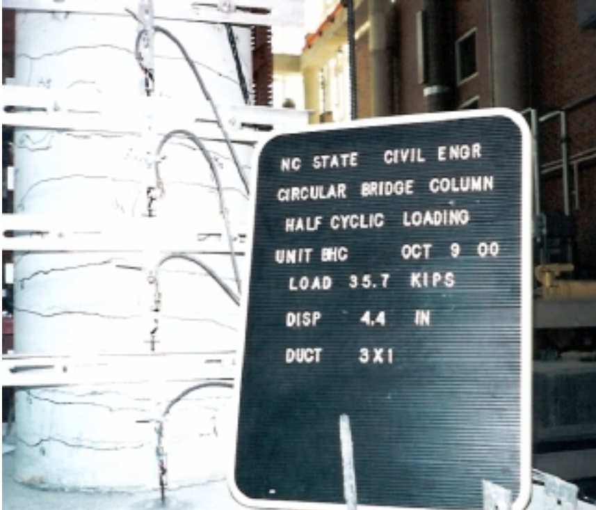
Figure 9.7 North Side of Specimen at Ductility 3 Cycle 1
