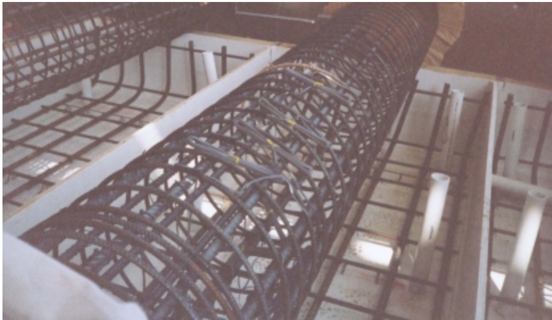
Figure 5.2 Column Reinforcement Spacing
