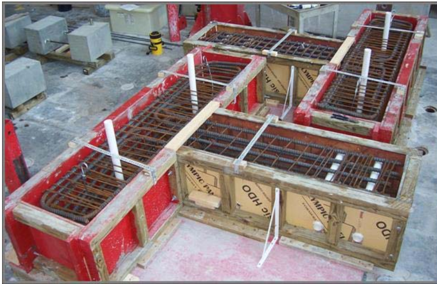
Figure 3.11. Forms, Reinforcement Steel, and Ducts - Two Specimens
