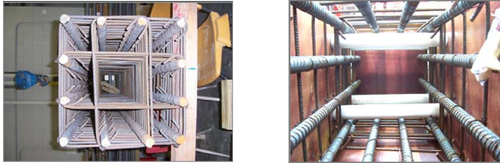
Figure 3.10. Steel Column Cross Sections – Ductile Shear Failure (Left), Brittle Shear Failure (Right)
