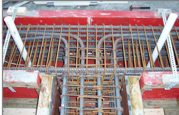
Figure 3.9. Reinforcement Steel – Column - Footing Connection
