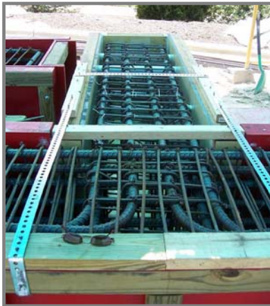
Figure 3.9. Reinforcement Steel – Column - Footing Connection
